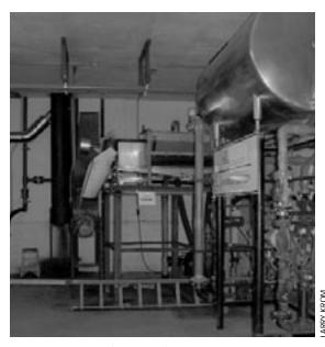
Heat exchanger tank (upper right) and solids separator. The heat exchanger transfers heat from the generator engine to the heating system for the barn and workshop. The solids separator recovers solids from the manure digestion process.
