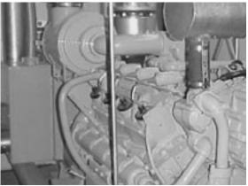
This generator engine uses gas from manure digestion as fuel. The generator produces about 120 kW of electricity.
