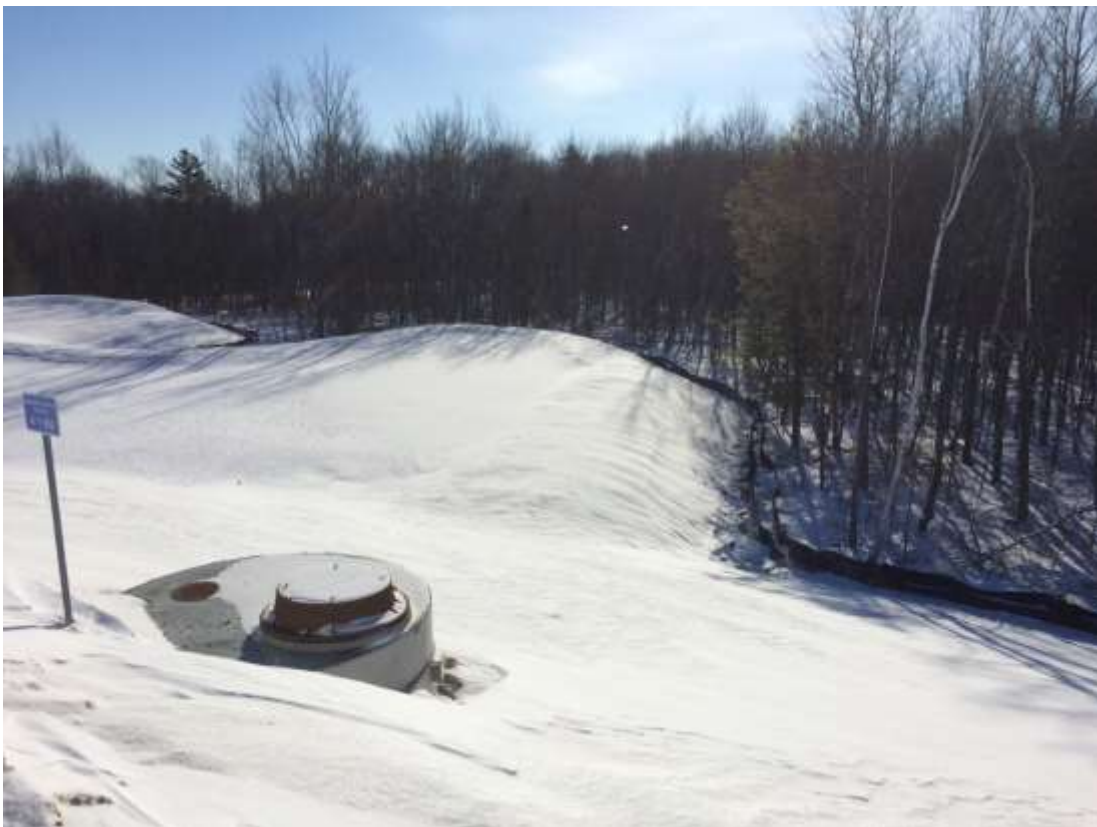
Photo 4 - Looking south from the south perimeter berm at storm water pond 3.
