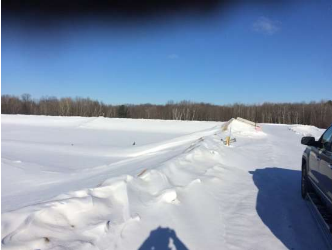
Photo 1 - WDS No. 3 looking north along perimeter berm at the Cell 1 Leachate Extraction Vault P1A
