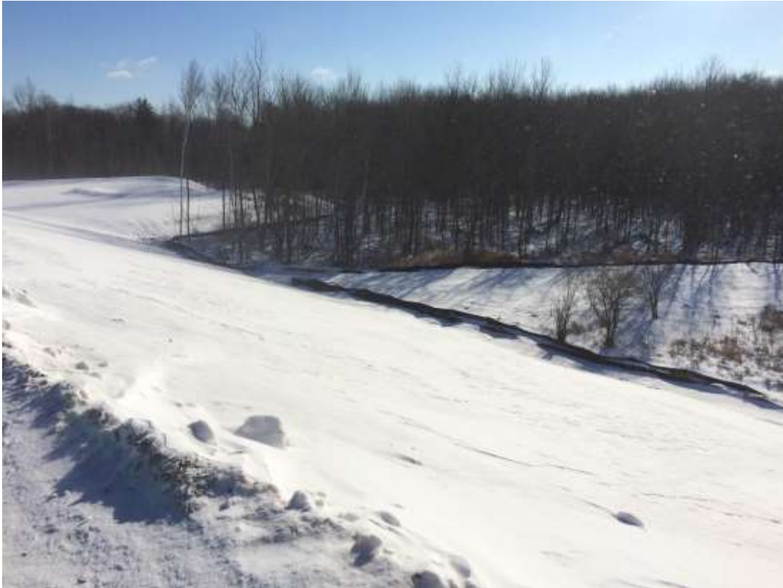
Photo 9 - WSD No. 3 looking at exterior slope of the South perimeter berm.
