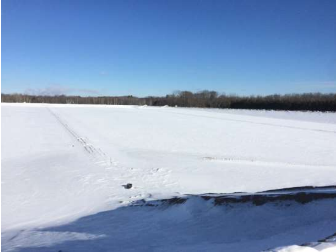
Photo 7 - WDS No. 3 looking north from South perimeter berm at the Cell 2
