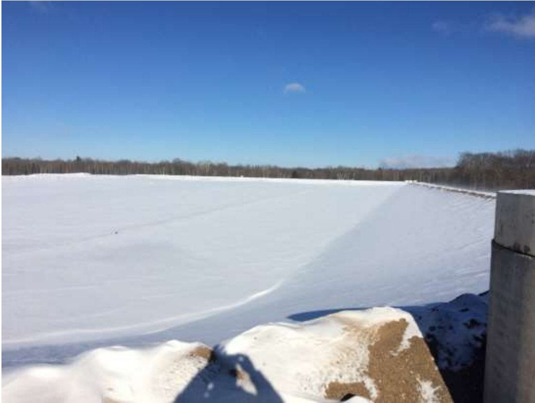
Photo 5 - WDS No. 3 looking north from South perimeter berm at the Cell 2.
