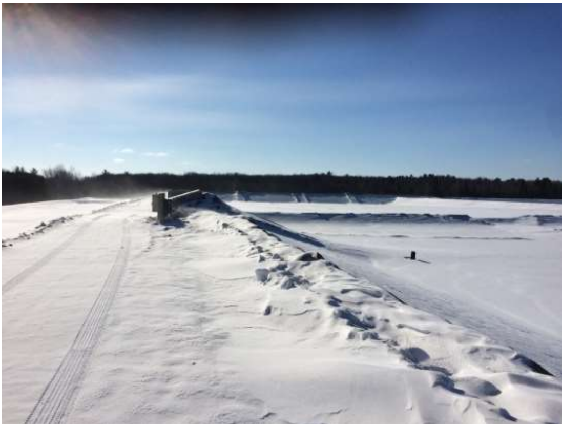
Photo 2 - WDS No. 3 looking south along perimeter berm at the Cell 1 Leachate Extraction Vault P1B.
