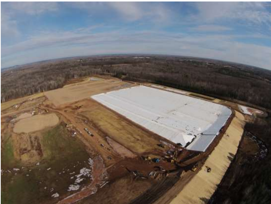
Photo 10 - WSD No. 3 Aerial Photo looking northeast, showing Cells 1 and 2 during construction (11/24/2015).
