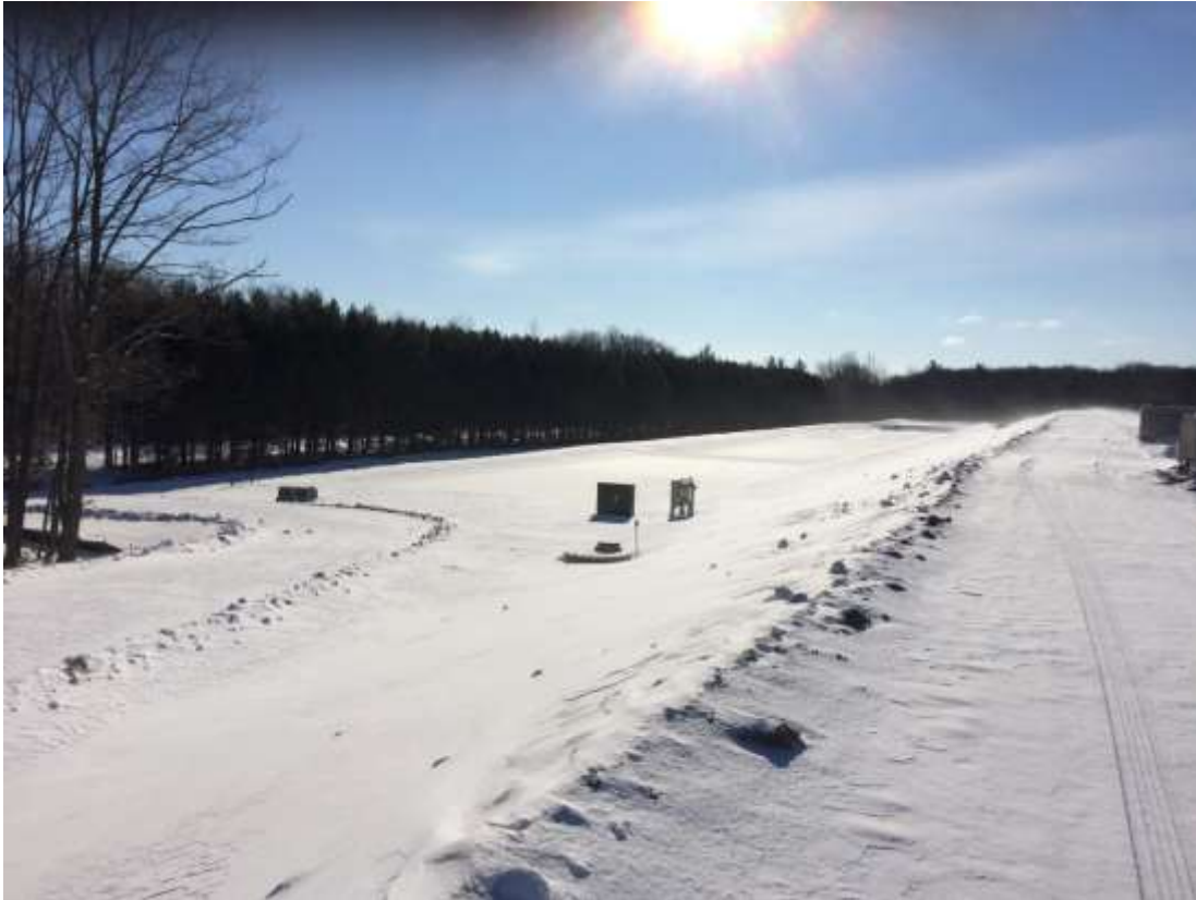
Photo 3 - WDS No. 3 looking south along perimeter berm at storm water pond 2 and emergency access.
