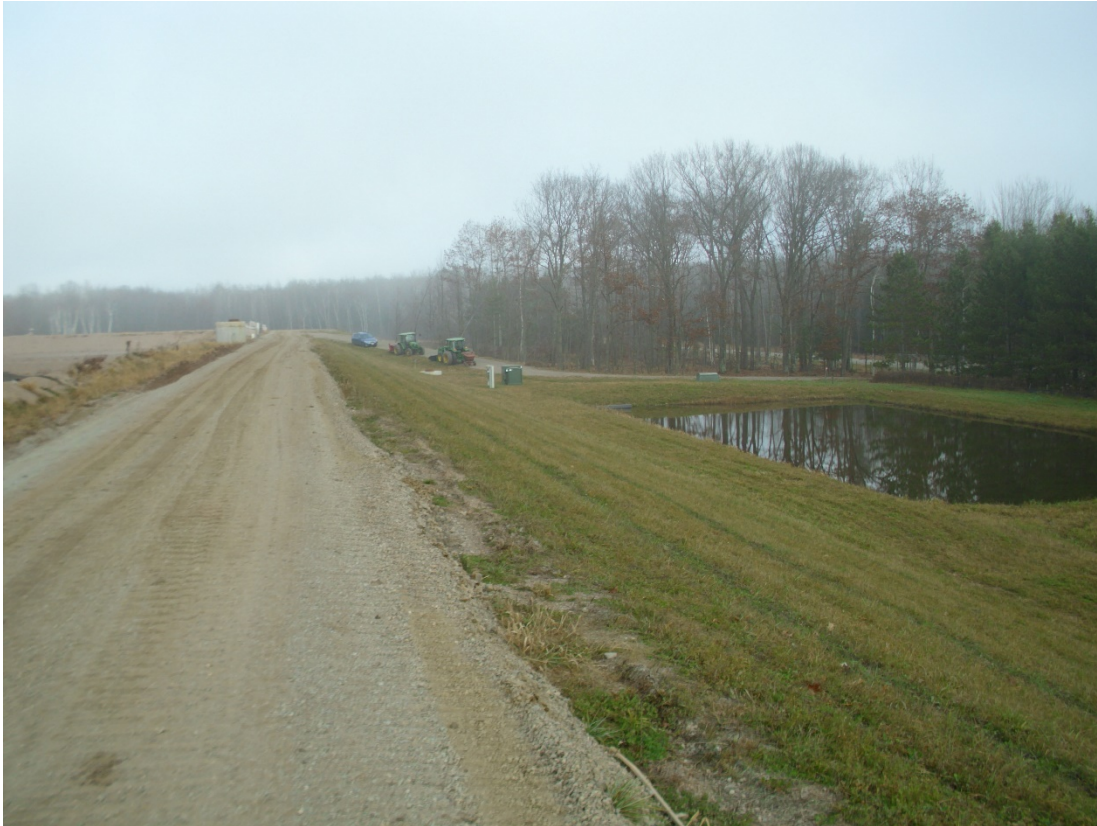
Photo 11 - WDS No. 3 looking north from South perimeter berm at the Cell 2
