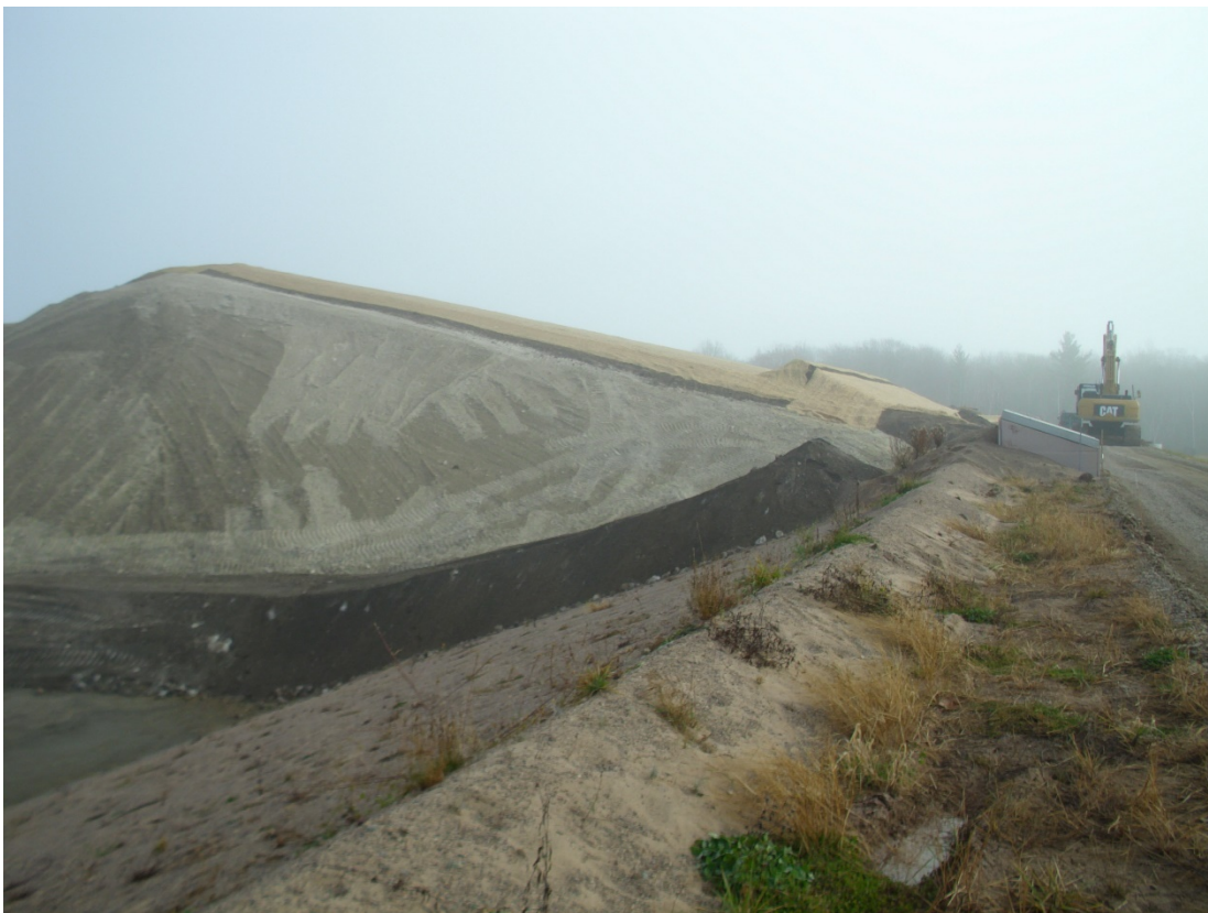
Photo 2 - Looking east along south perimeter berm at Leachate Extraction Vault P2B.
