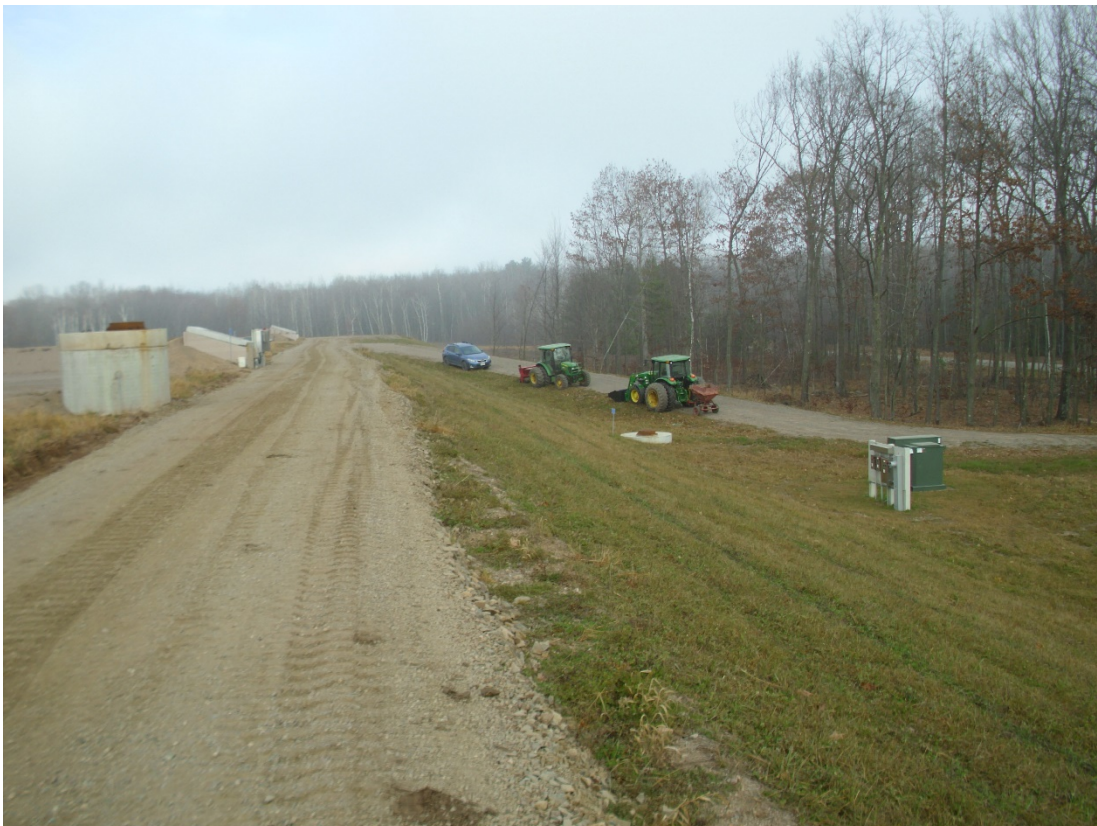
Photo 12 - WDS No. 3 looking Leachate Extraction Vault P2B.
