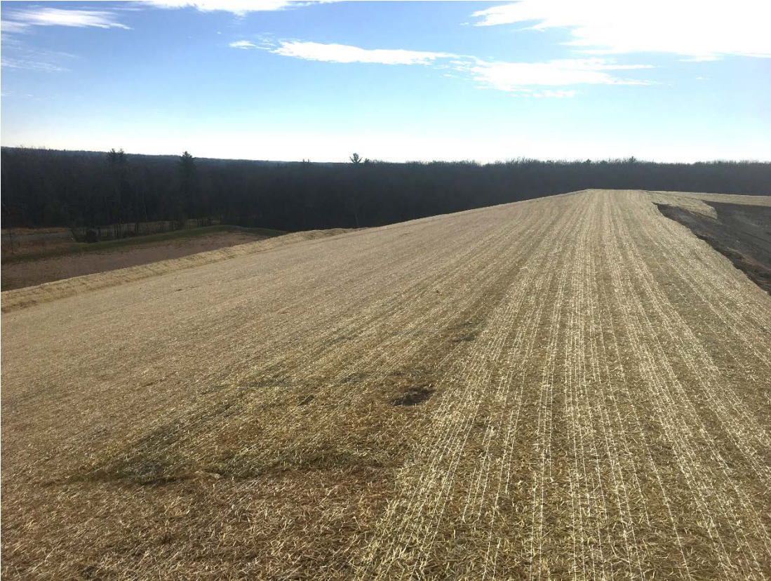
Photo 9 - Looking south along top of Cell 2 partial final cover.
