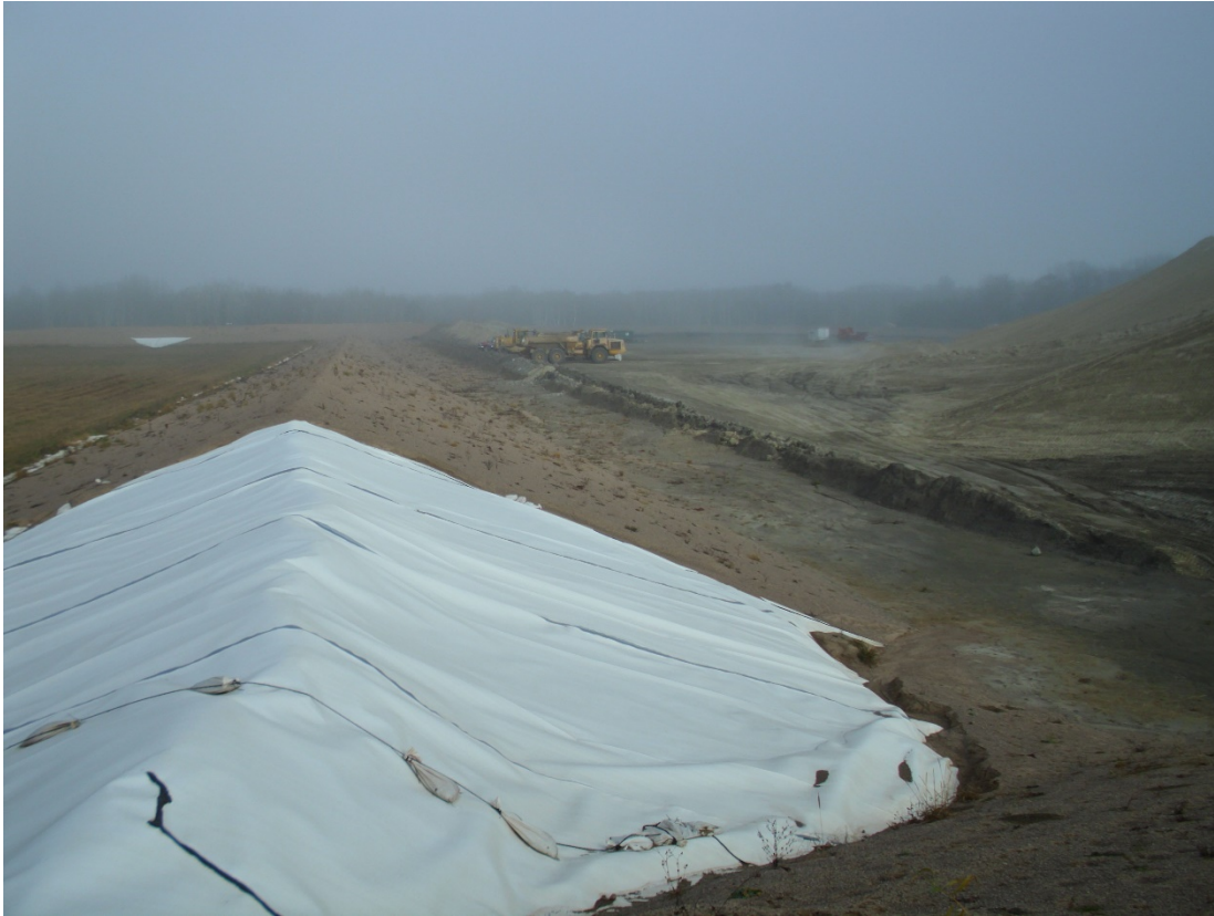
Photo 1 - Looking north along Cell 2-3 intercell berm.
