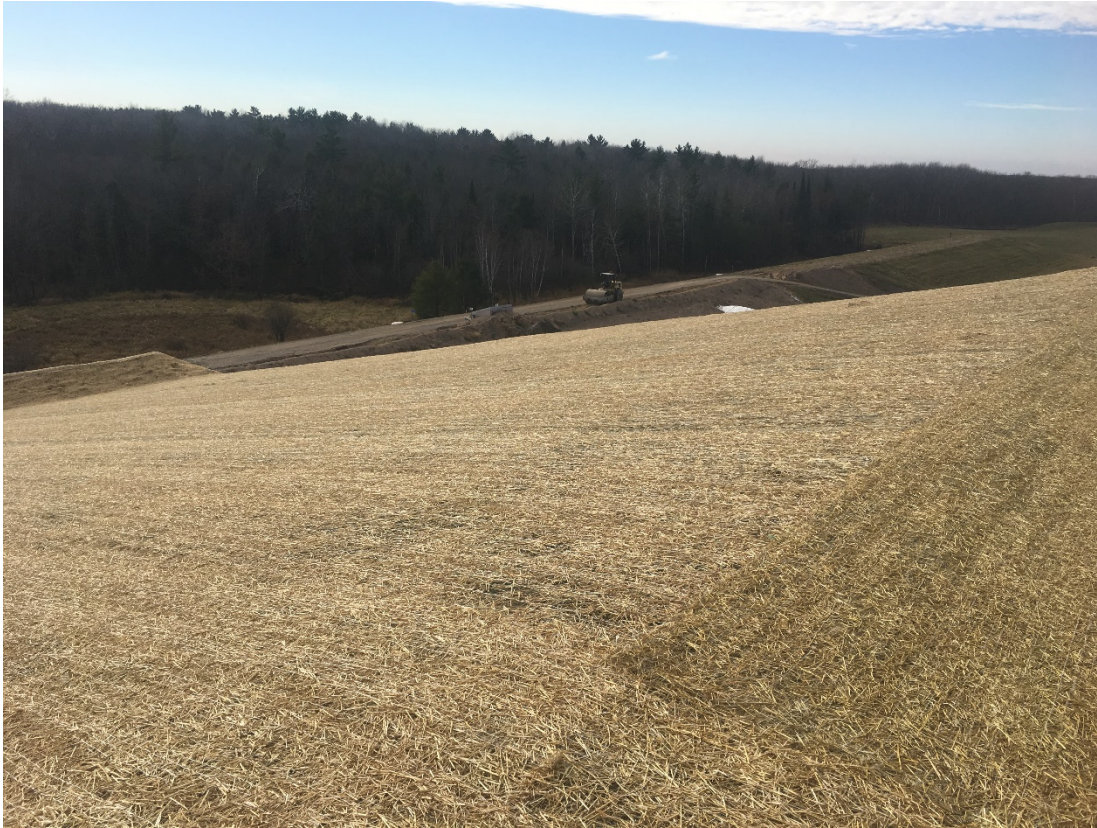
Photo 3 - Looking southwest from top of Cell 2 partial final cover.
