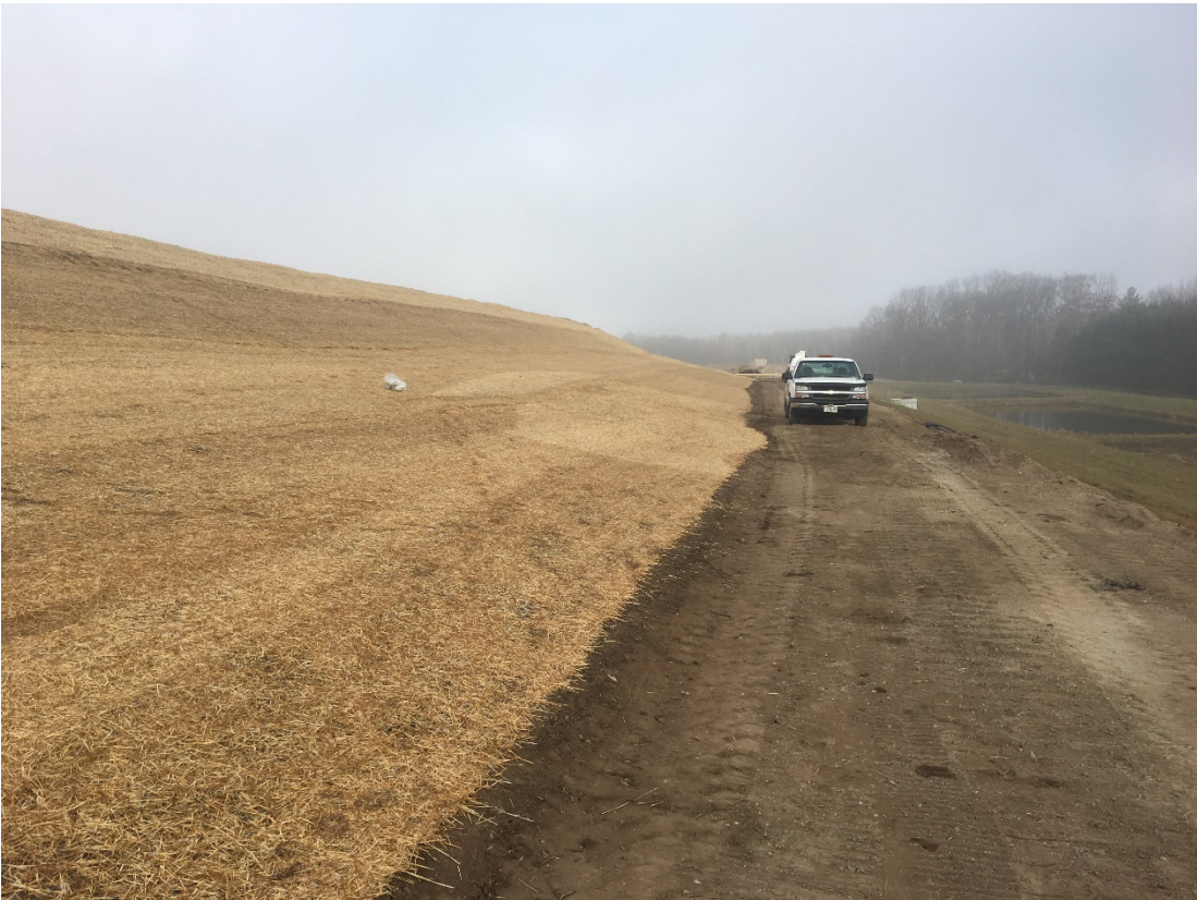
Photo 10 – Looking north along east perimeter berm of Cell 2.
