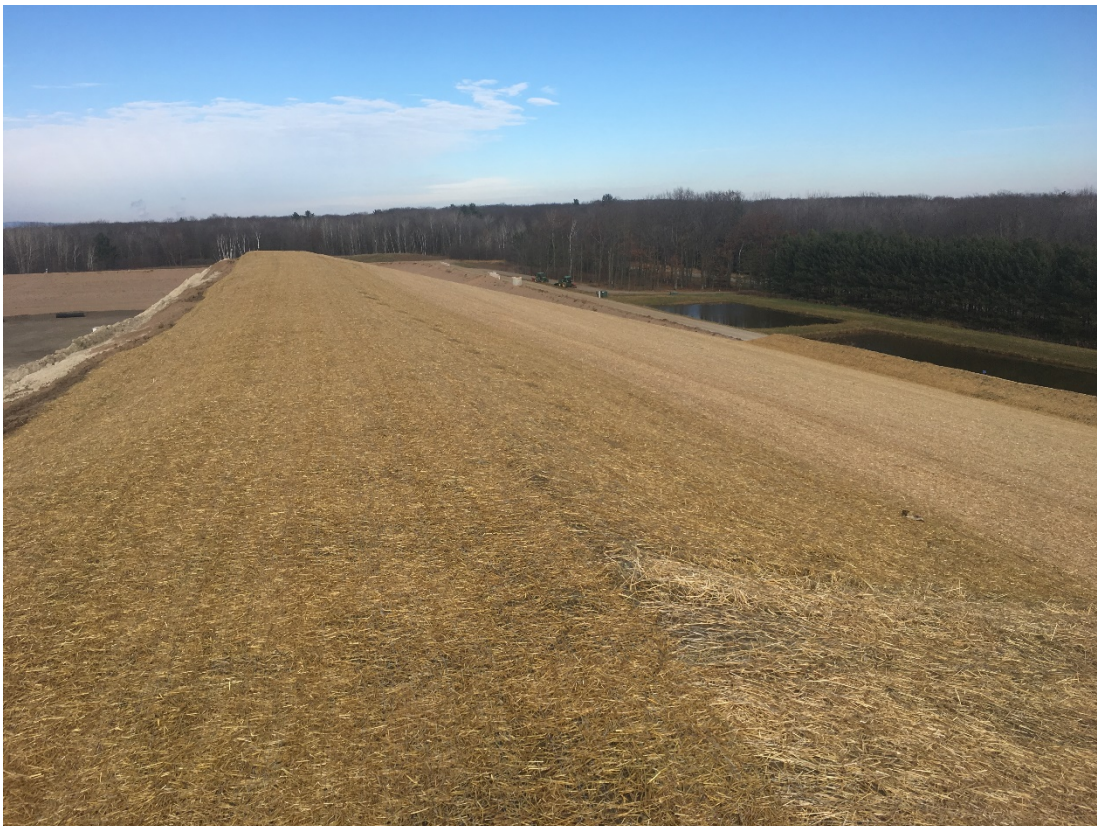
Photo 8 - Looking north along top of Cell 2 partial final cover.
