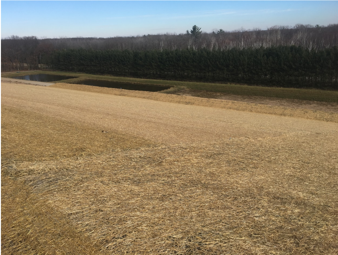
Photo 7 - Looking east from top of Cell 2 partial final cover at Stormwater Basin 2.
