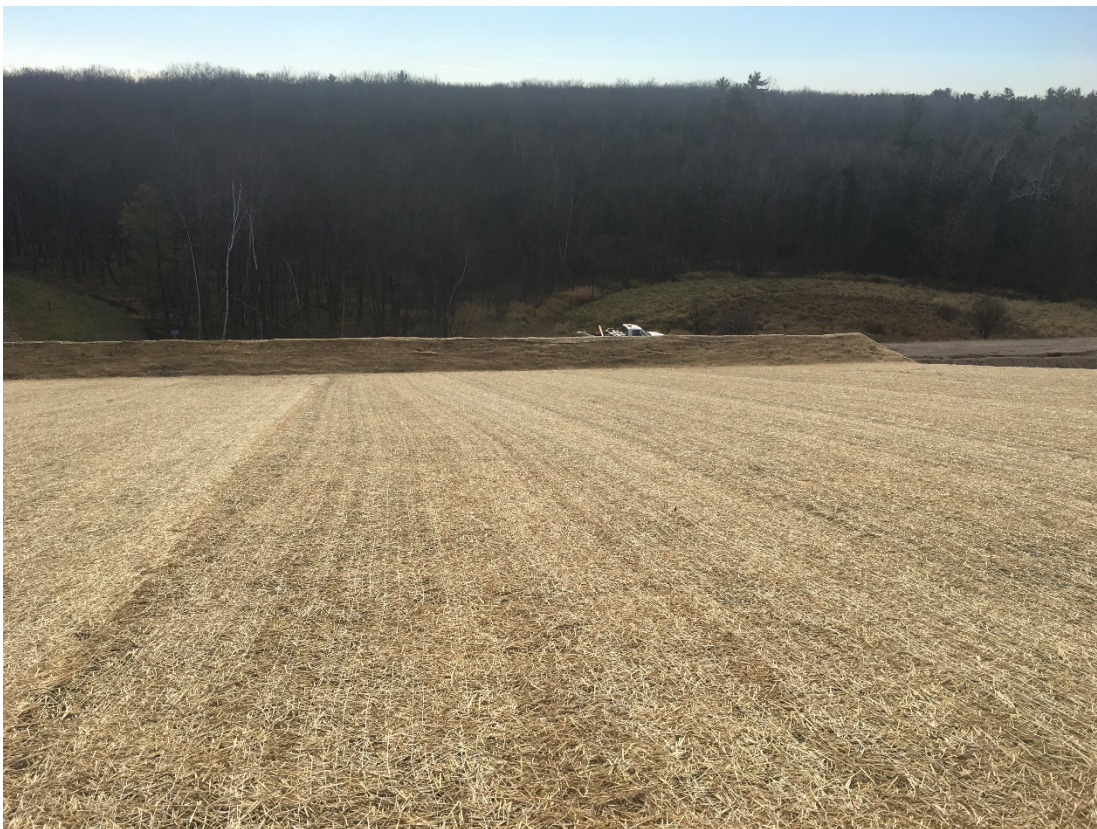
Photo 4 - Looking south from top of Cell 2 partial final cover.
