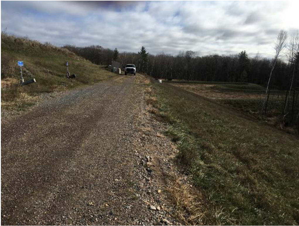
Photo 5 – Along south perimeter berm near Leachate Extraction Vault P2B.
