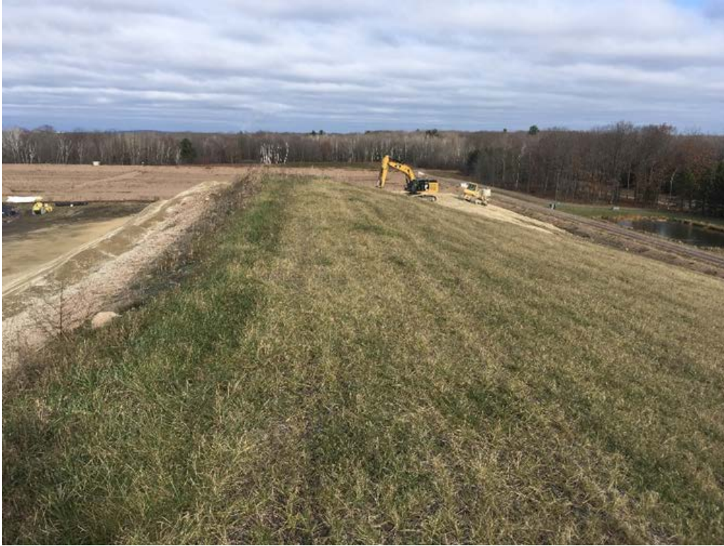
Photo 9 - Along top of Cell 2 partial final cover.
