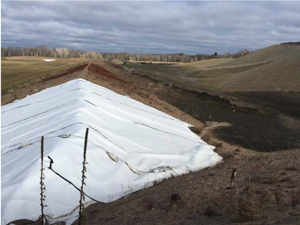
Photo 4 - Along cell 2-3 intercell berm.
