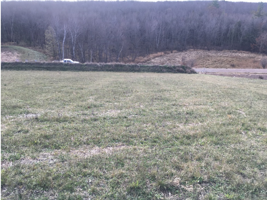
Photo 6 – From top of Cell 2 partial final cover towards south perimeter berm.
