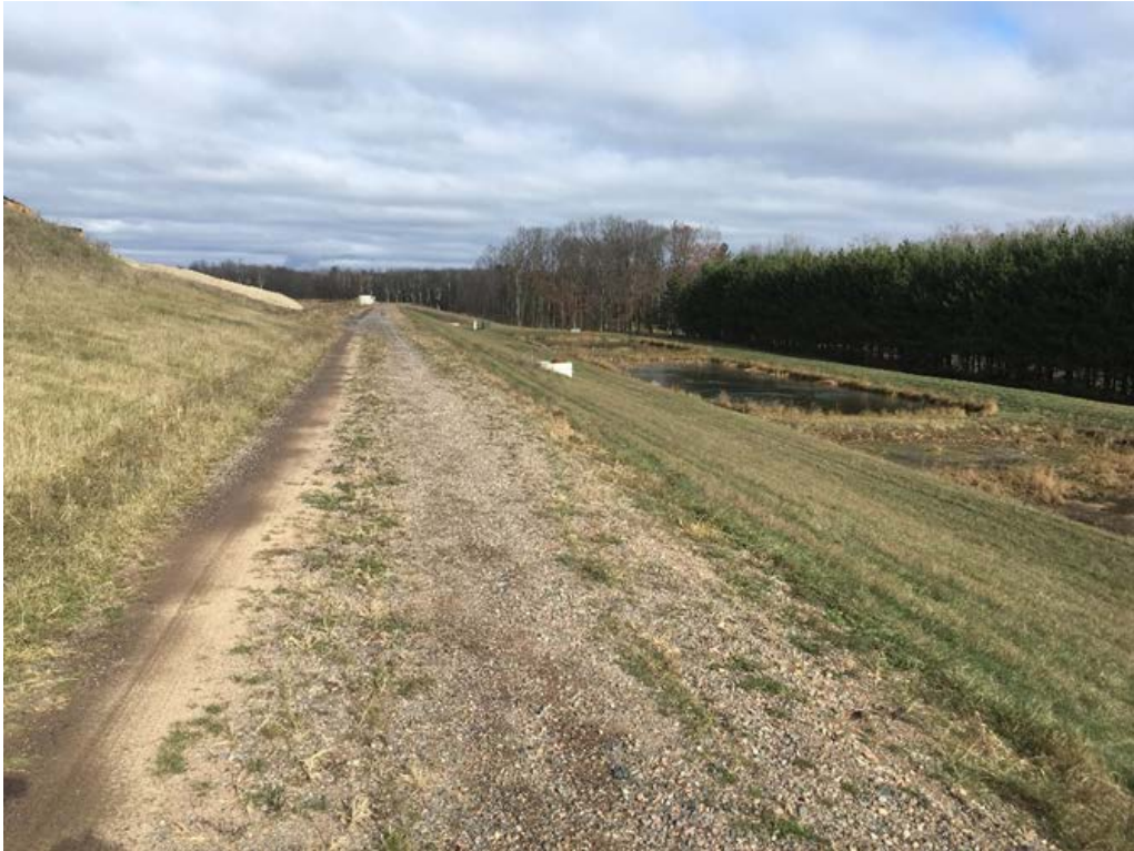
Photo 10 – Along east perimeter berm of Cell 2.
