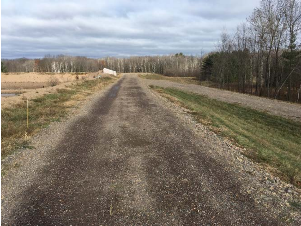
Photo 12 - WDS No. 3 looking Leachate Extraction Vault P2B.
