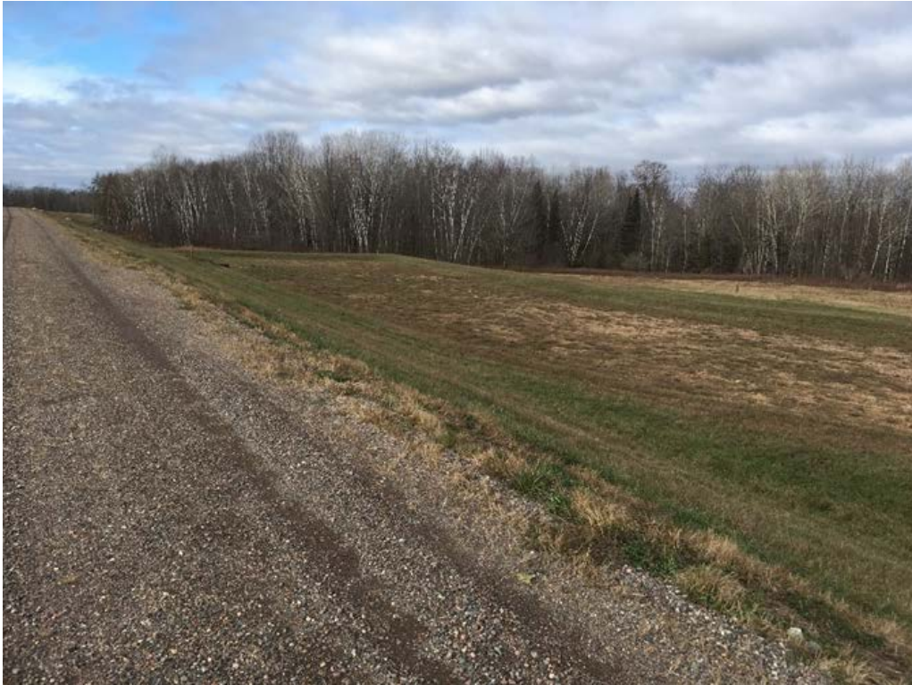
Photo 14 - Looking west along the north perimeter berm of Cells 1.
