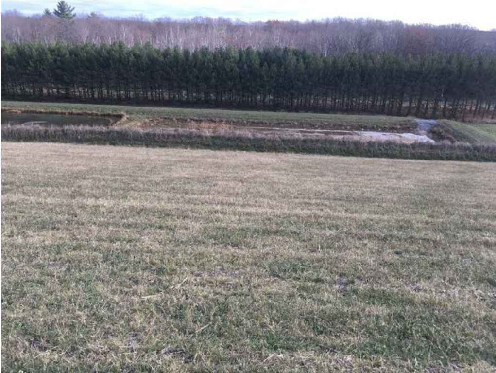
Photo 8 - From top of Cell 2 partial final cover at Stormwater Basin 2.
