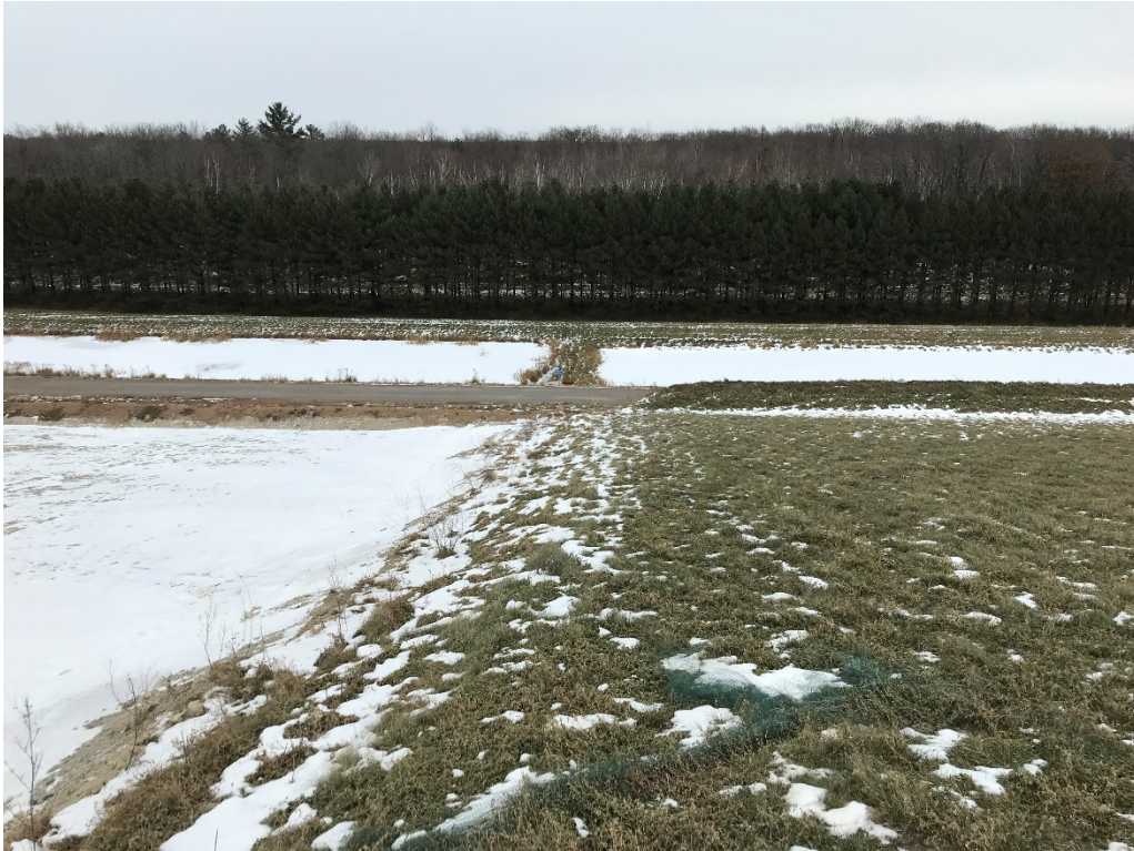
Photo 10 – From top of Cell 2 partial final cover at Stormwater Basin 2.
