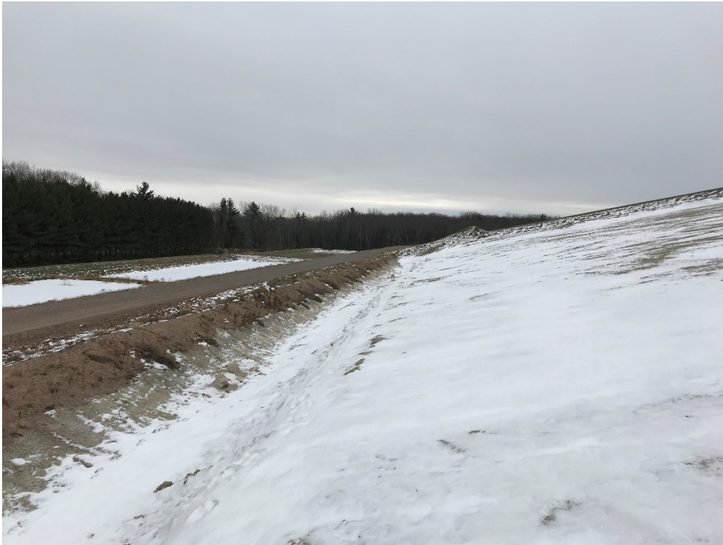
Photo 13 - Looking north to the east showing stormwater control ditch.
