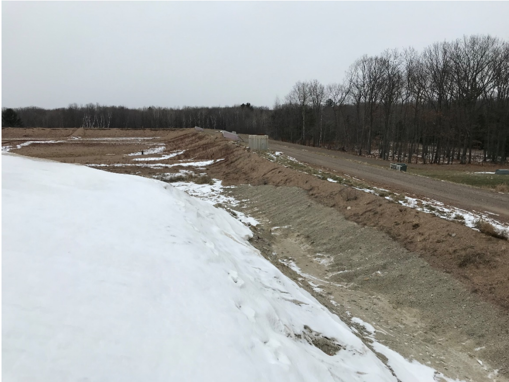
Photo 14 - Looking north to the west towards Cell 1 showing stormwater control ditch..
