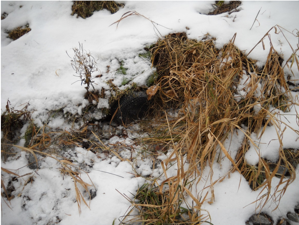
Photo 1 - Westernmost gradient control pipe along south perimeter berm.
