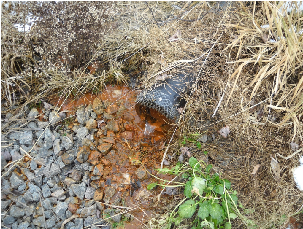
Photo 3 - Easternmost gradient control pipe along south perimeter berm.
