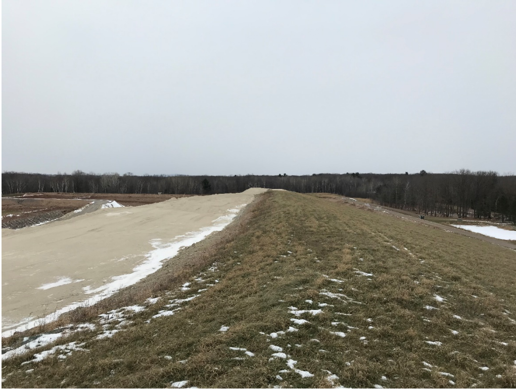
Photo 9 - Along top of Cell 2 partial final cover.
