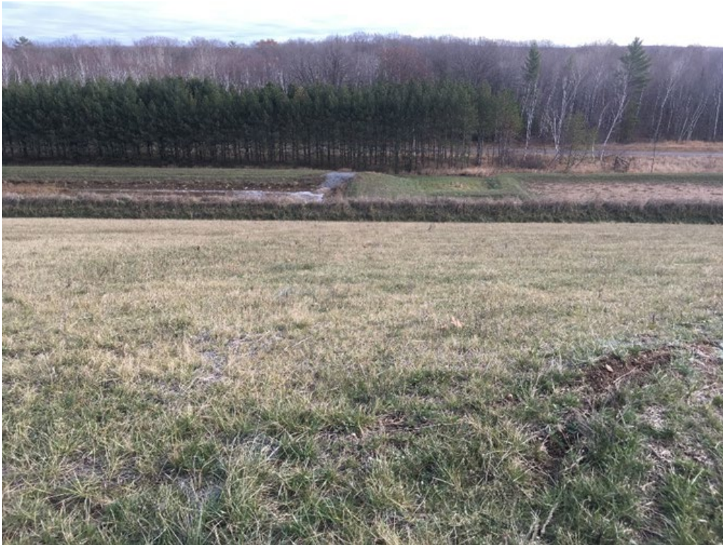
Photo 7 - From top of Cell 2 partial final cover at Stormwater Basin 2 and Stormwater Basin 3
