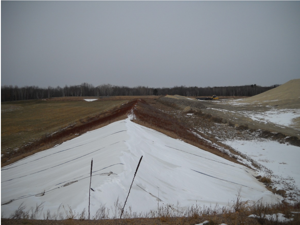
Photo 4 - Along cell 2-3 intercell berm.
