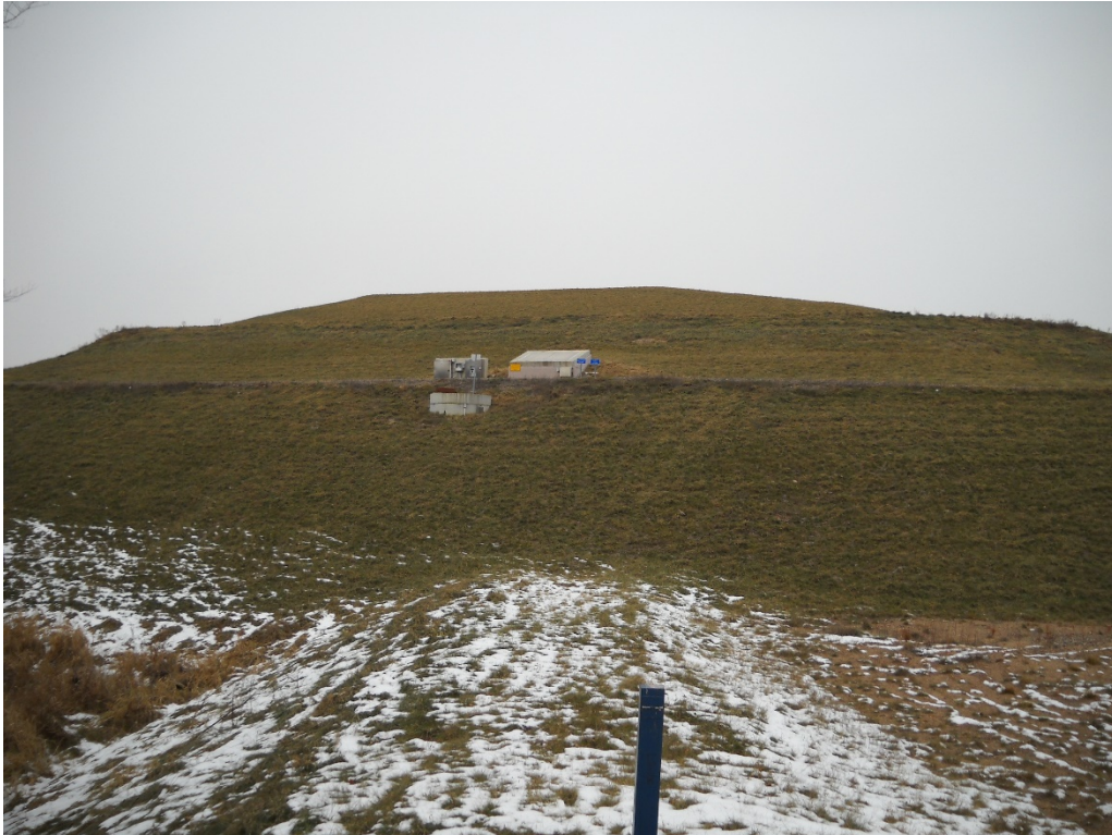
Photo 6 – Looking at the south perimeter slope from the Stormwater Basin 3
