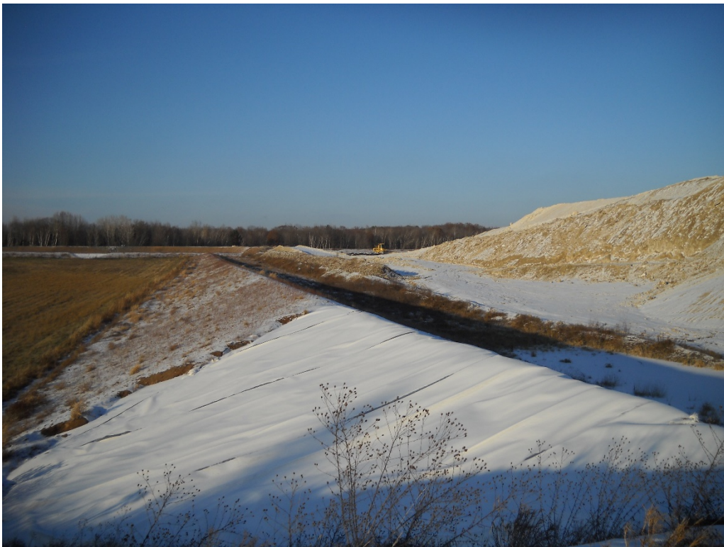
Photo 2 - Along cell 2-3 intercell berm.
