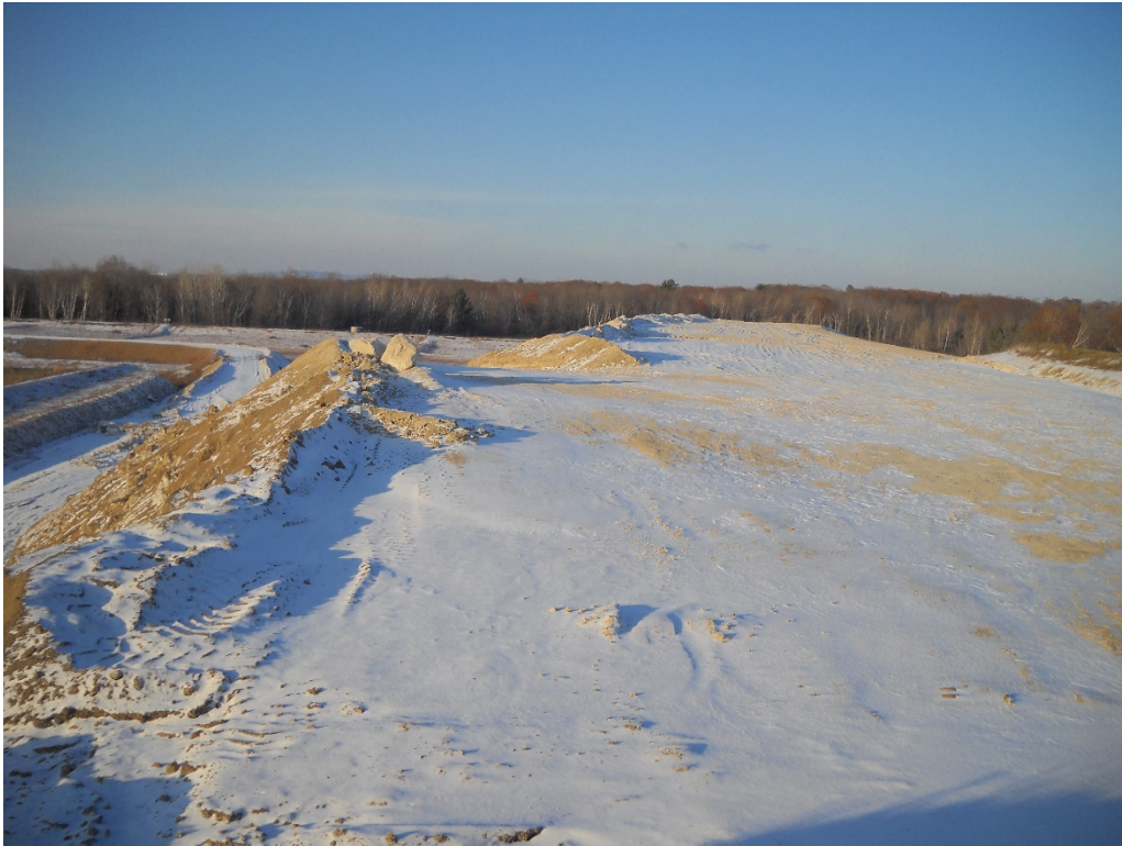
Photo 1 – Looking north showing the active filling area.
