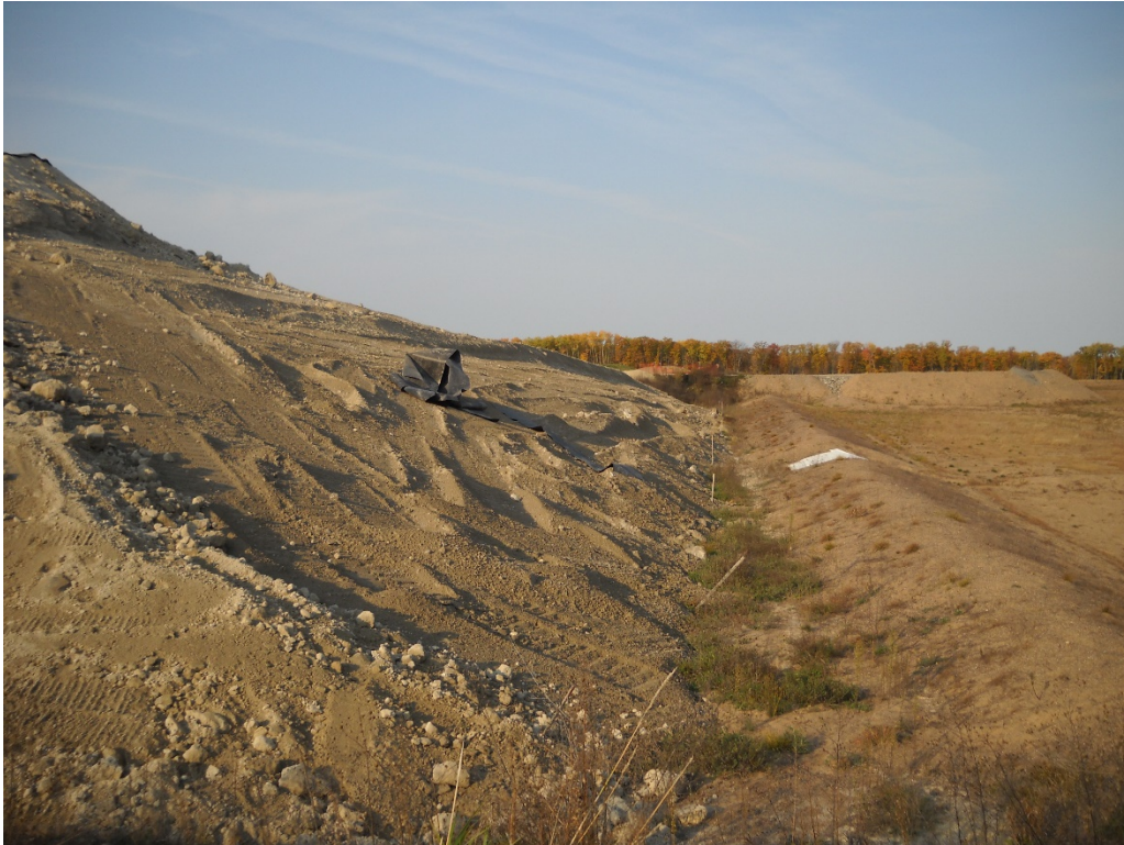
Photo 10 - Looking at north ash slope in Cell 2.
