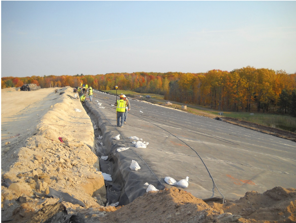
Photo 9 - Looking at covered east slope in Cell 2 towards Cell 1.
