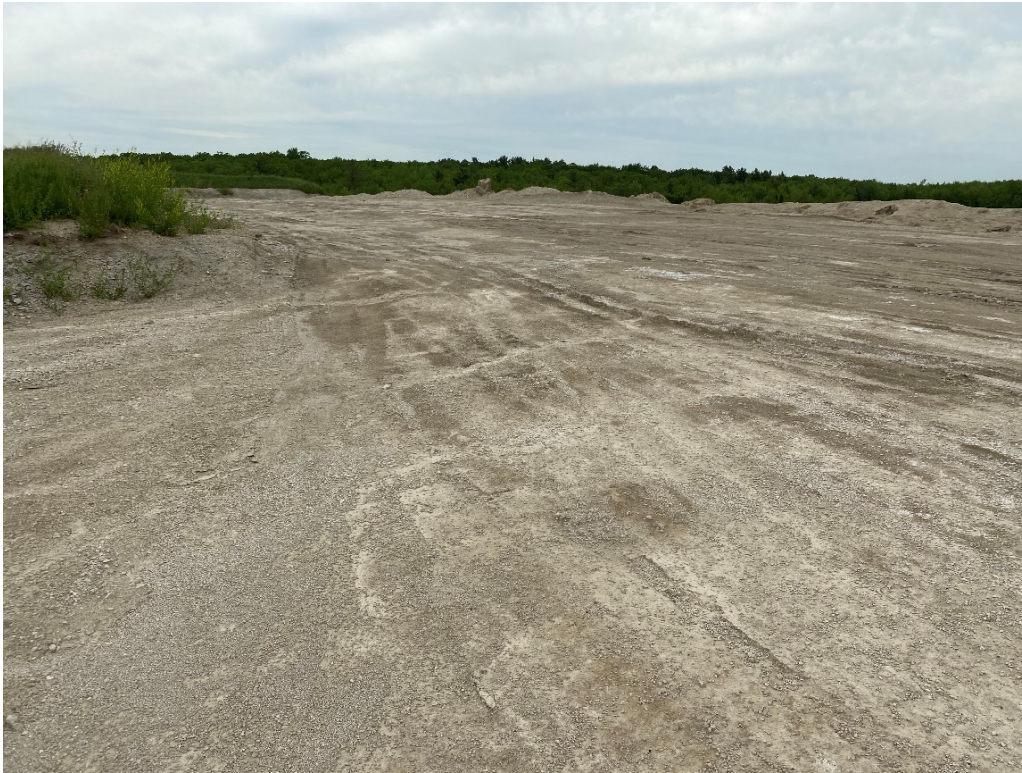
Photo 1 – Looking north showing the active filling area.
