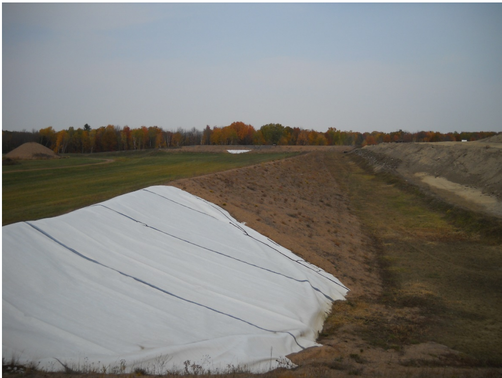
Photo 2 - Along cell 2-3 intercell berm.
