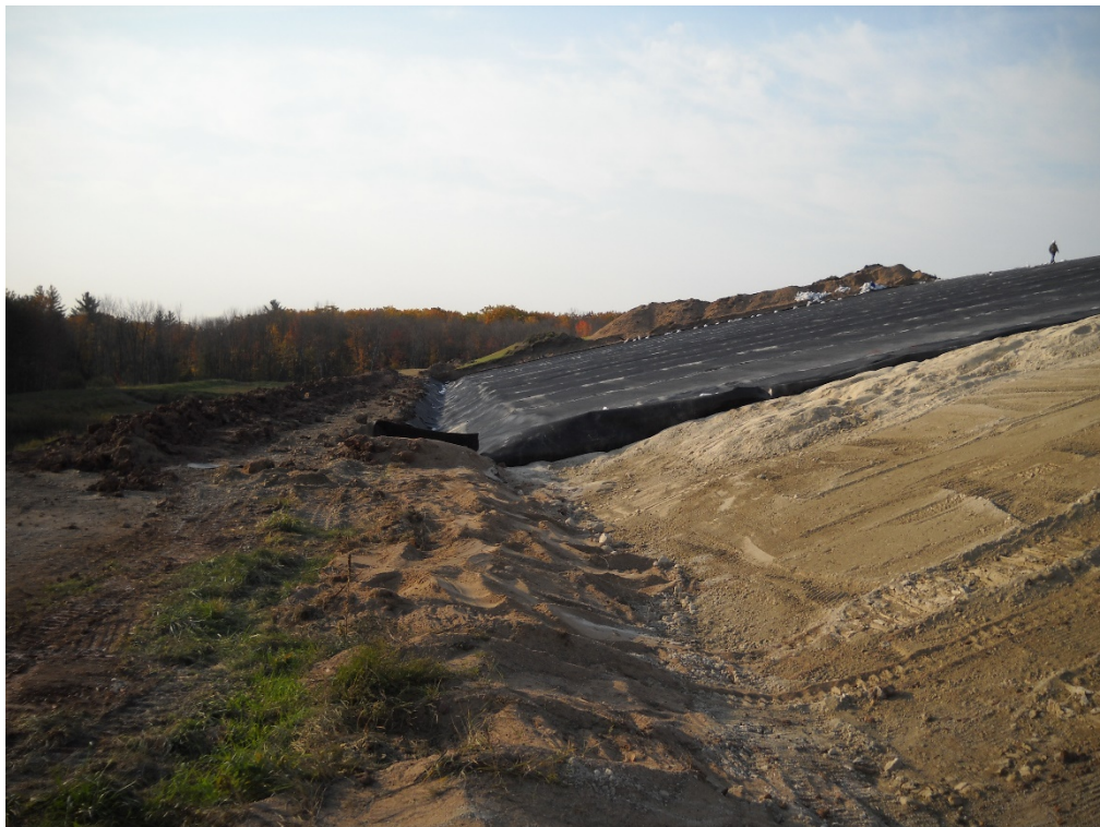
Photo 8 – Looking south to final cover and active filling area.
