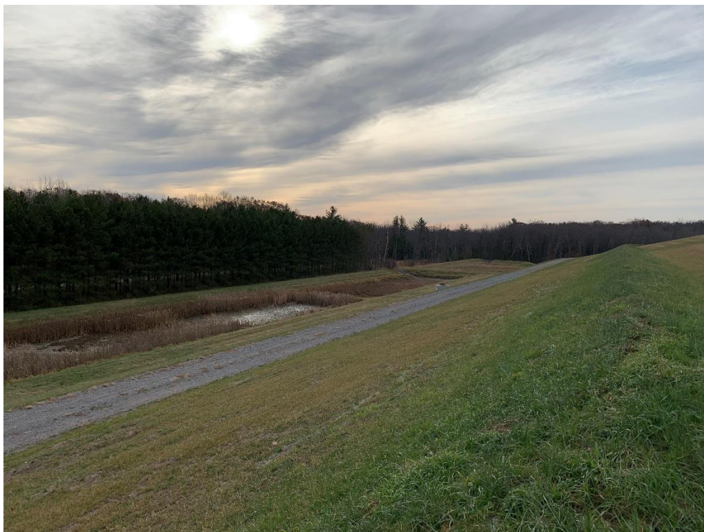
Photo 6 - From top of Cell 2 partial final cover at Stormwater Basin 2.
