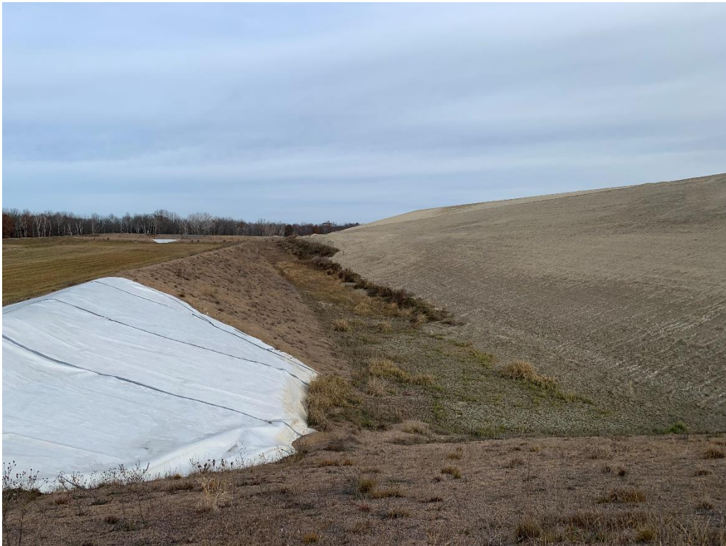
Photo 2 - Along Cell 2-3 intercell berm.
