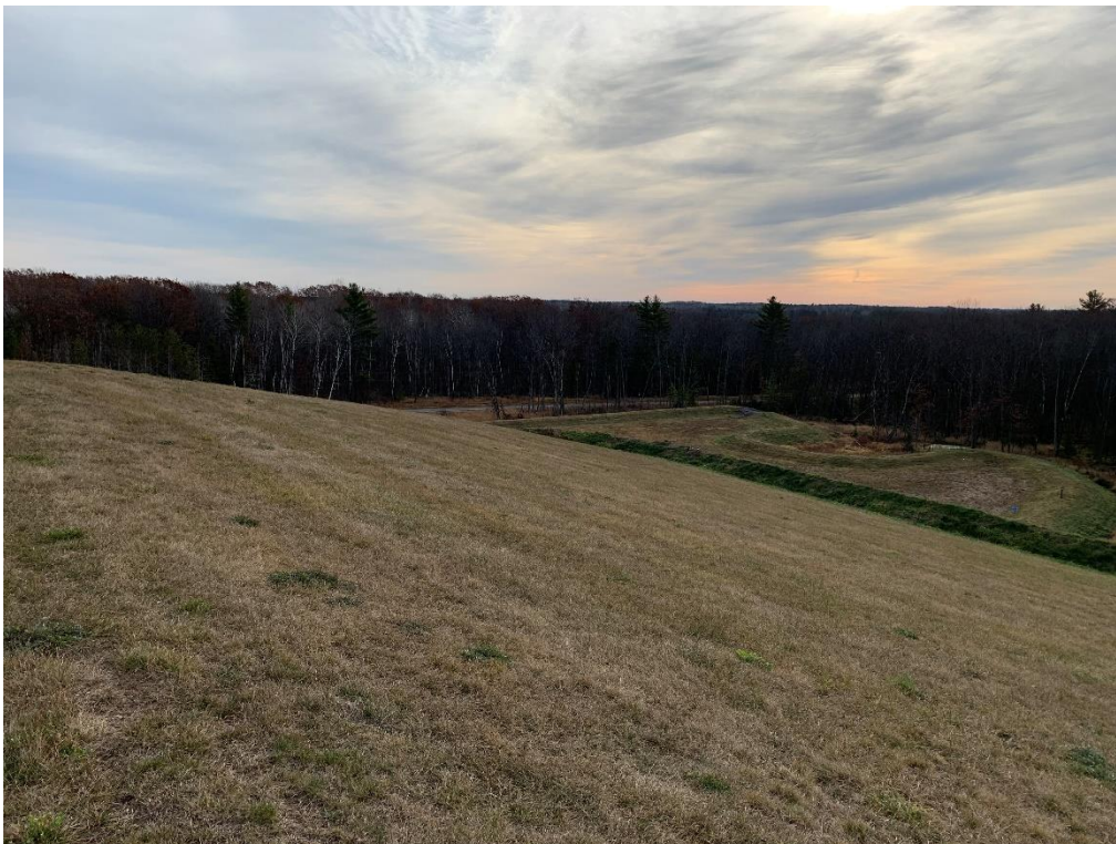
Photo 4 – Looking at the south perimeter slope from the top of the final cover.
