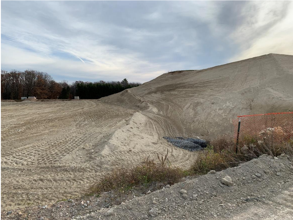
Photo 10 - Looking at north ash slope in Cell 2 and frost protection layer in Cell 1.
