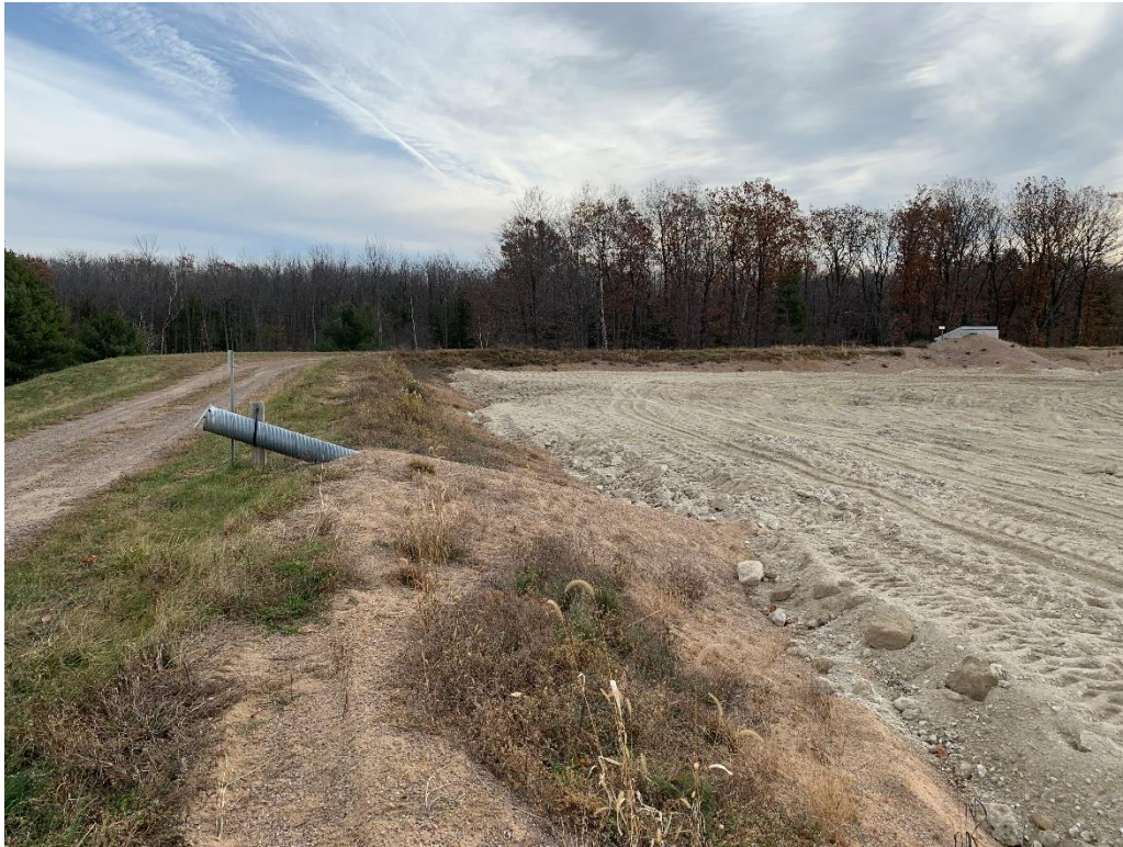
Photo 9 - Looking east at Cell 1 perimeter slopes showing the frost protection layer.
