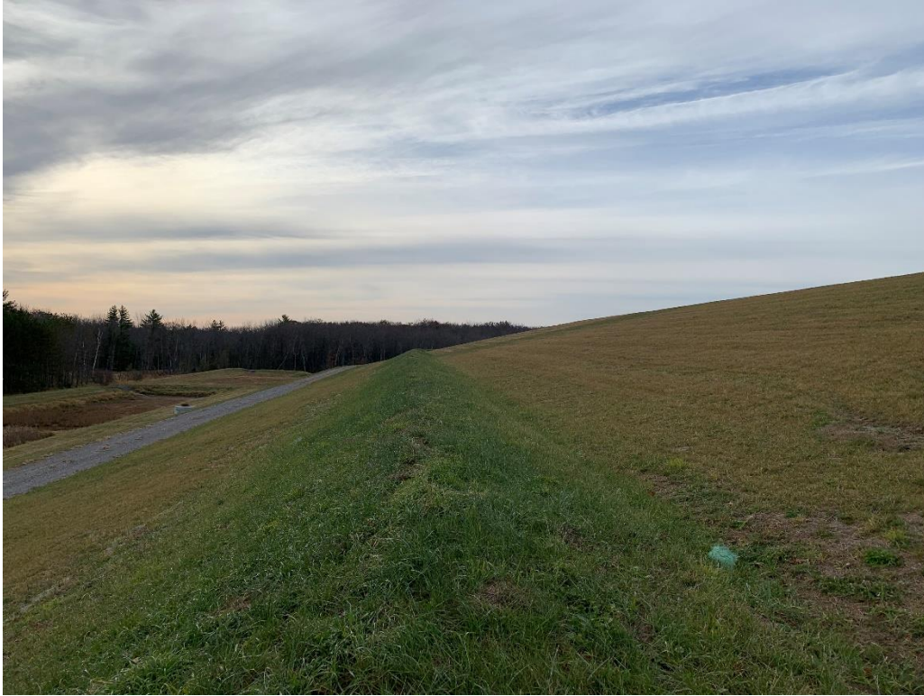
Photo 11 - Looking south at the east stormwater control ditch.
