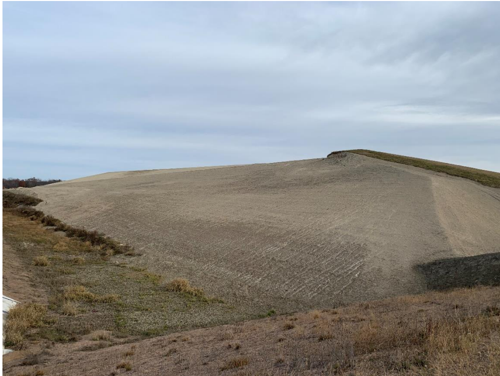
Photo 3 – Along south perimeter berm near Leachate Extraction Vault P2B.
