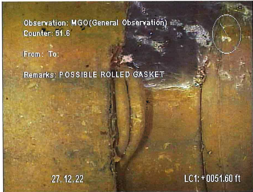
Date: 2022/12/27 Distance: 51.6 Ft Obs: General Observation Comments: POSSIBLE ROLLED GASKET
