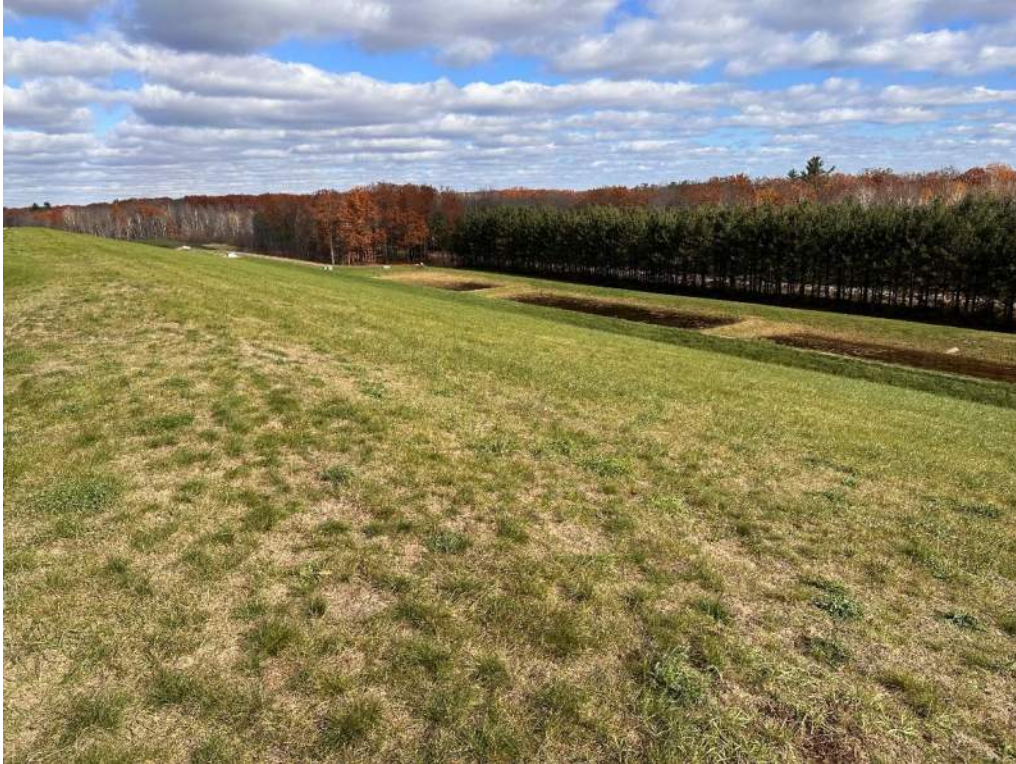
Photo No. 5 – Stormwater Basin 2 east of Cell 2.
