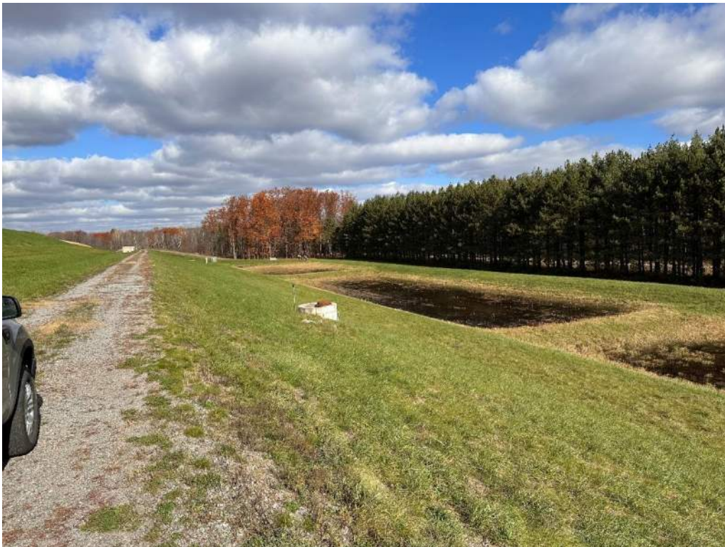
Photo No. 6 – Stormwater Basin 2.
