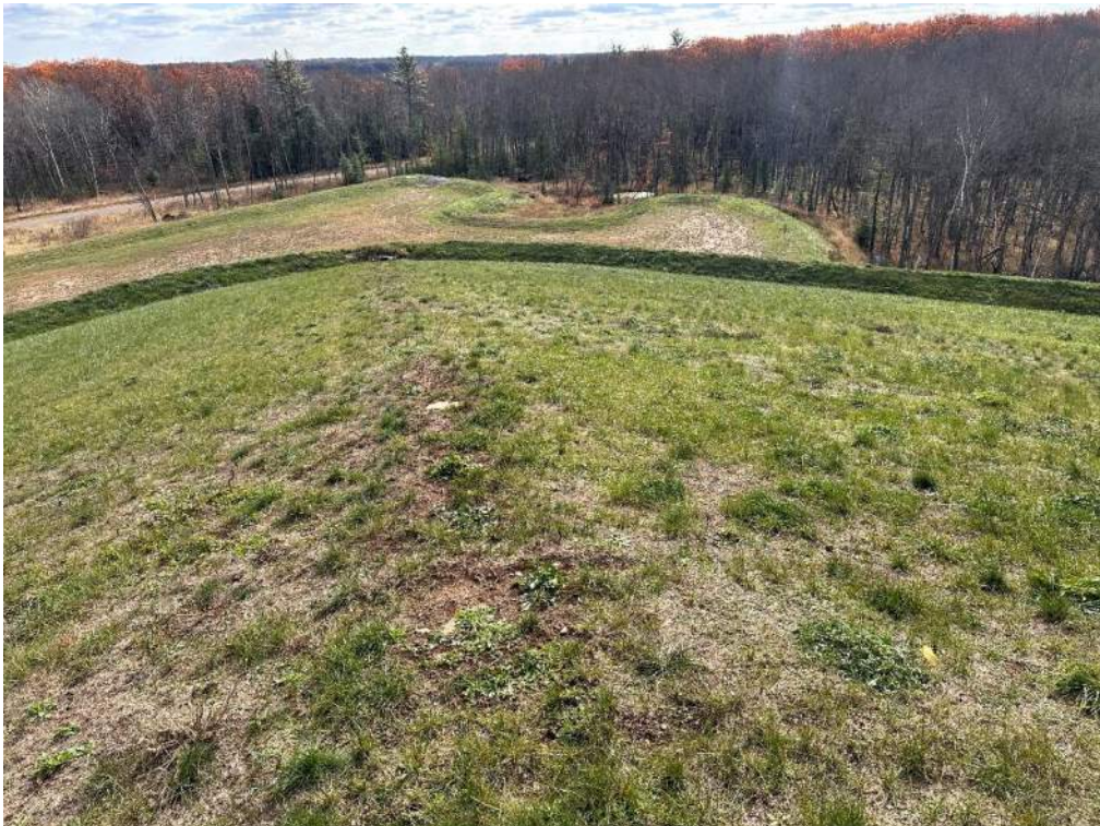
Photo No. 4 – Cell 2 south and east slope and stormwater diversion berm.
