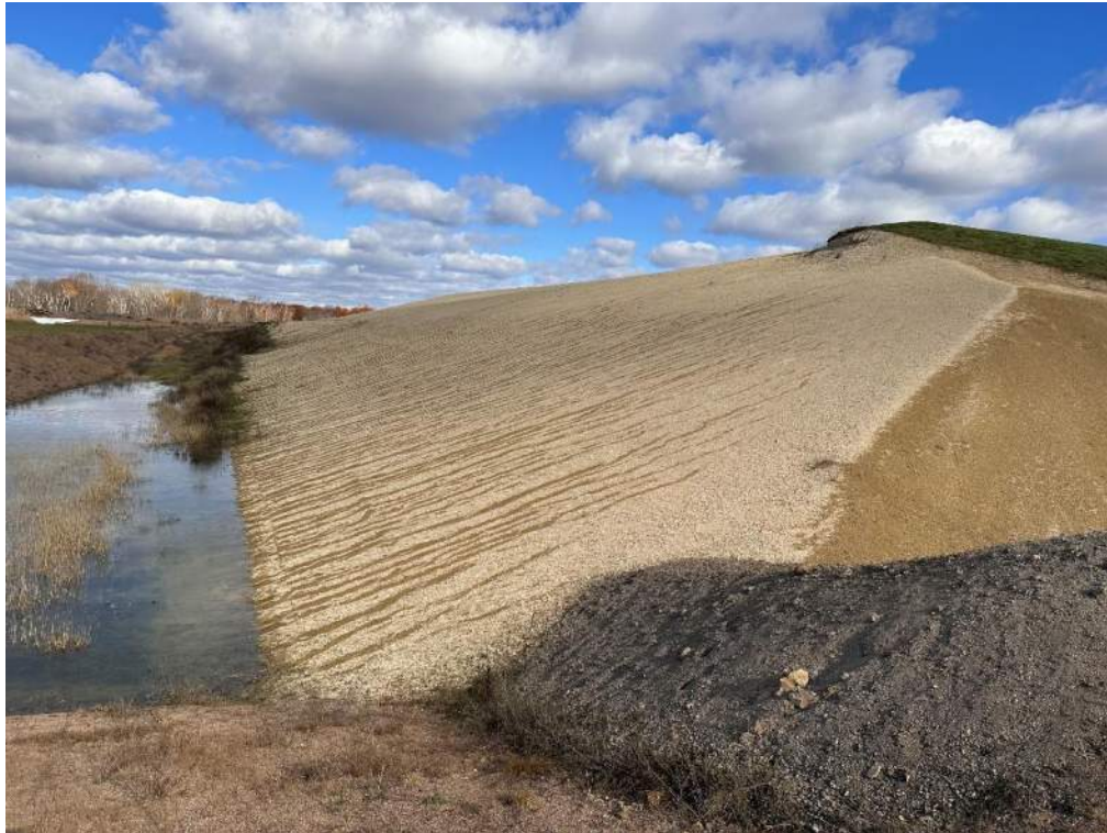
Photo No. 3 – Cell 2 west slope.
