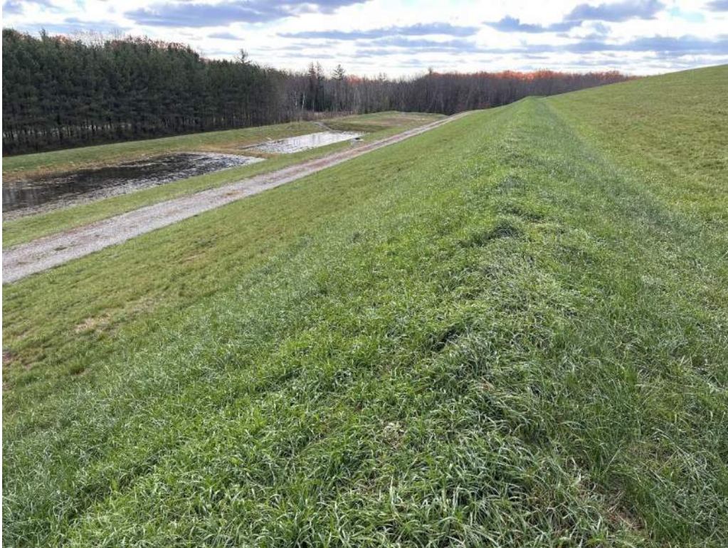
Photo No. 11 – Looking south at the Cell 2 east stormwater control ditch.
