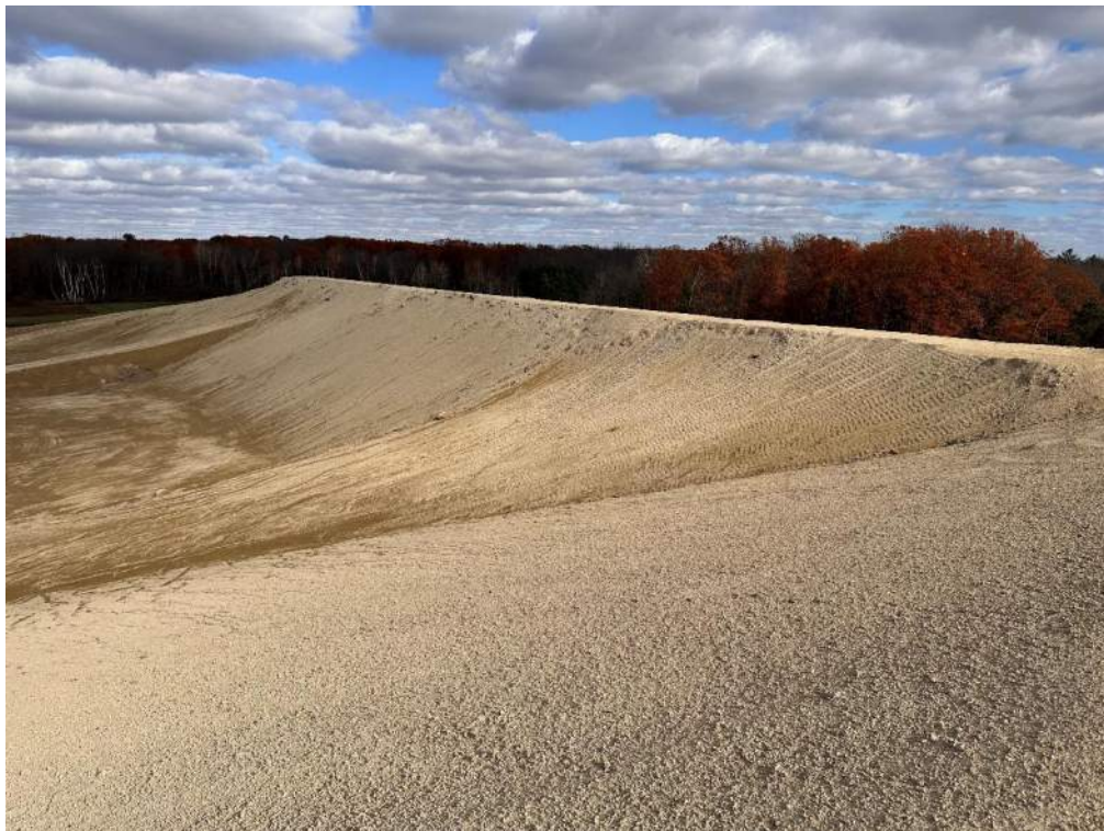
Photo No. 8 – Looking northeast to the Cell 1 active filling area and the east slope prepared for final cover.
