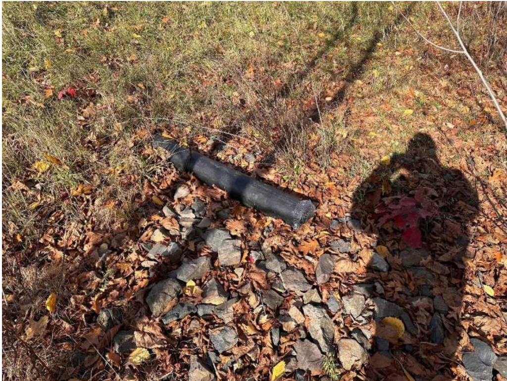
Photo No. 15 – Cell 1 gradient control outlet pipe.
