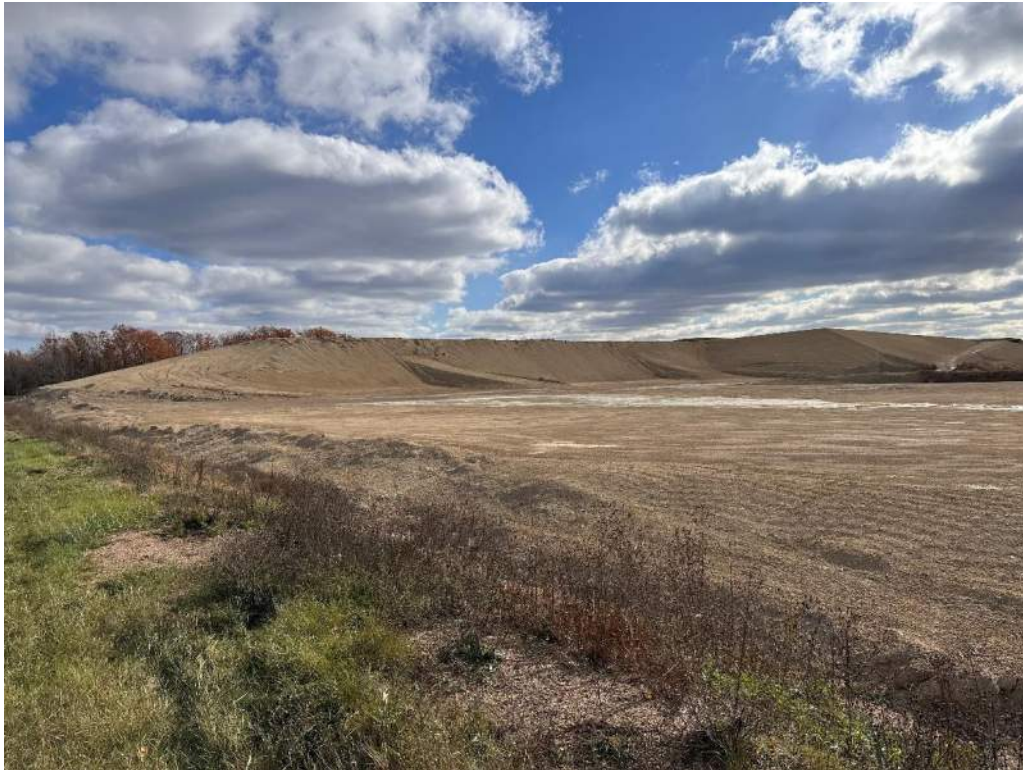
Photo No. 7 – Active filling area in Cell 1, looking east.
