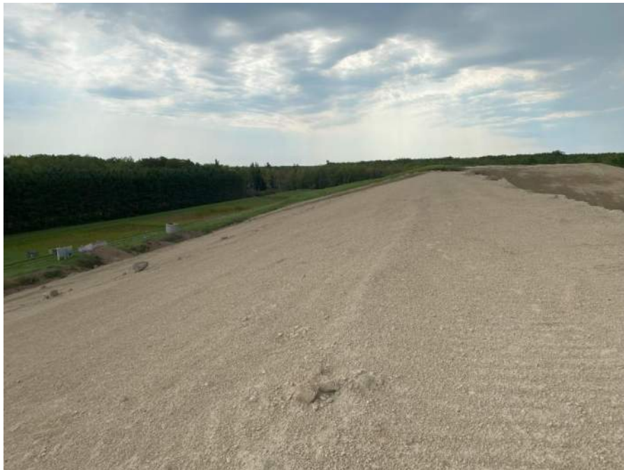
Photo No. 8 – Looking south on the Cell 1 active filling area and the east slope prepared for final cover.
