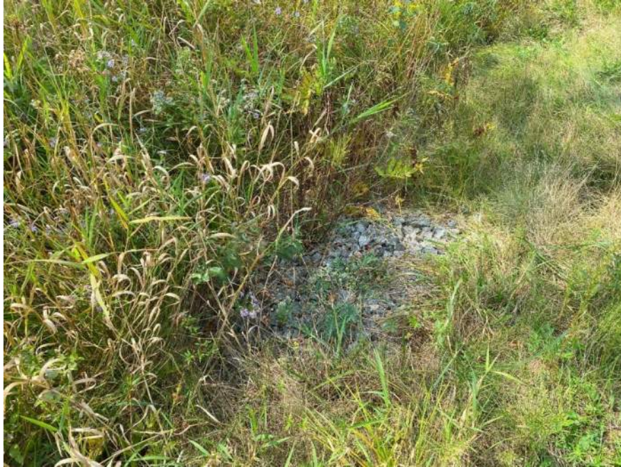
Photo No. 13 – Cell 2 gradient control outlet pipe.
