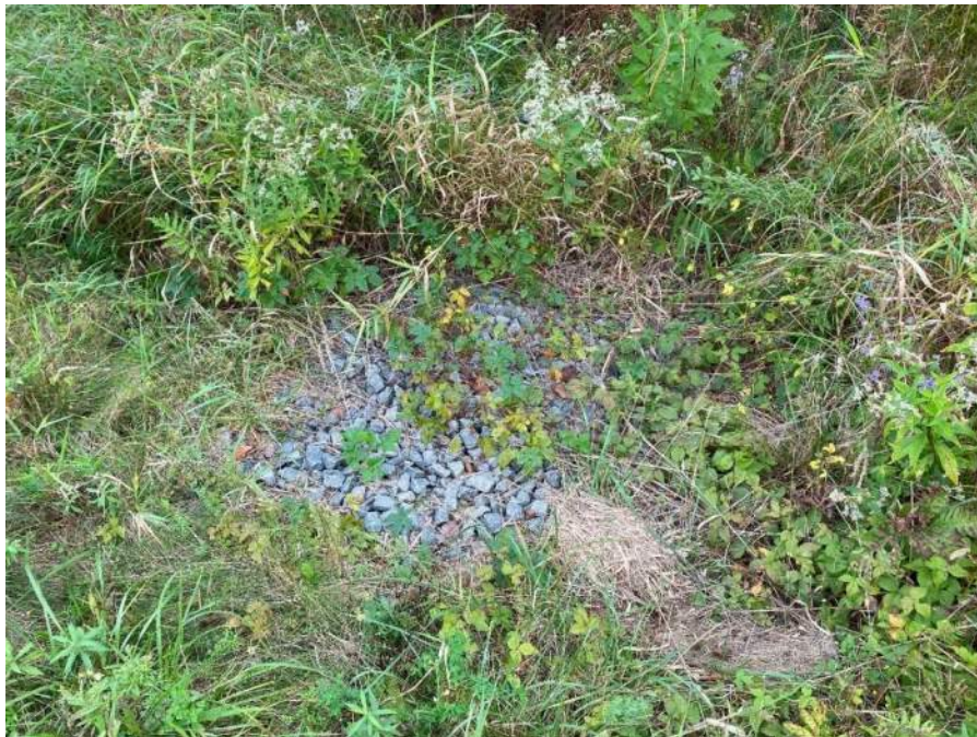
Photo No. 14 – Cell 2 gradient control outlet pipe.
