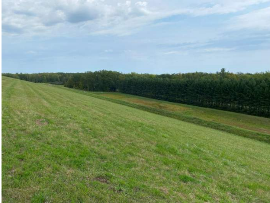
Photo No. 5 – Stormwater Basin 2 east of Cell 2.
