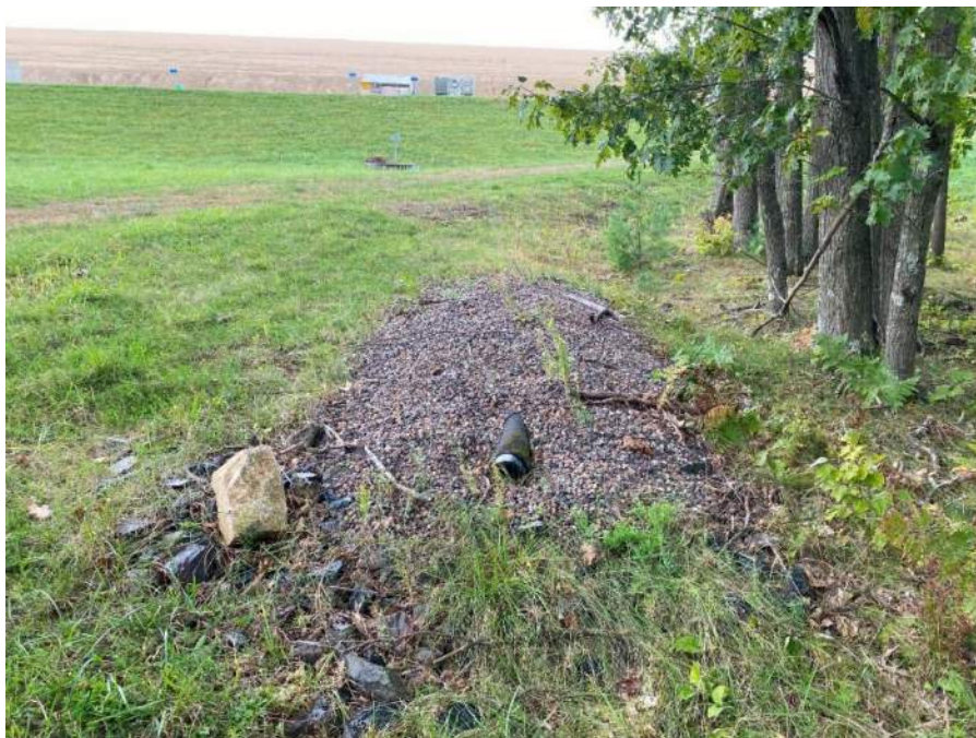
Photo No. 16 – Cell 1 gradient control outlet pipe.
