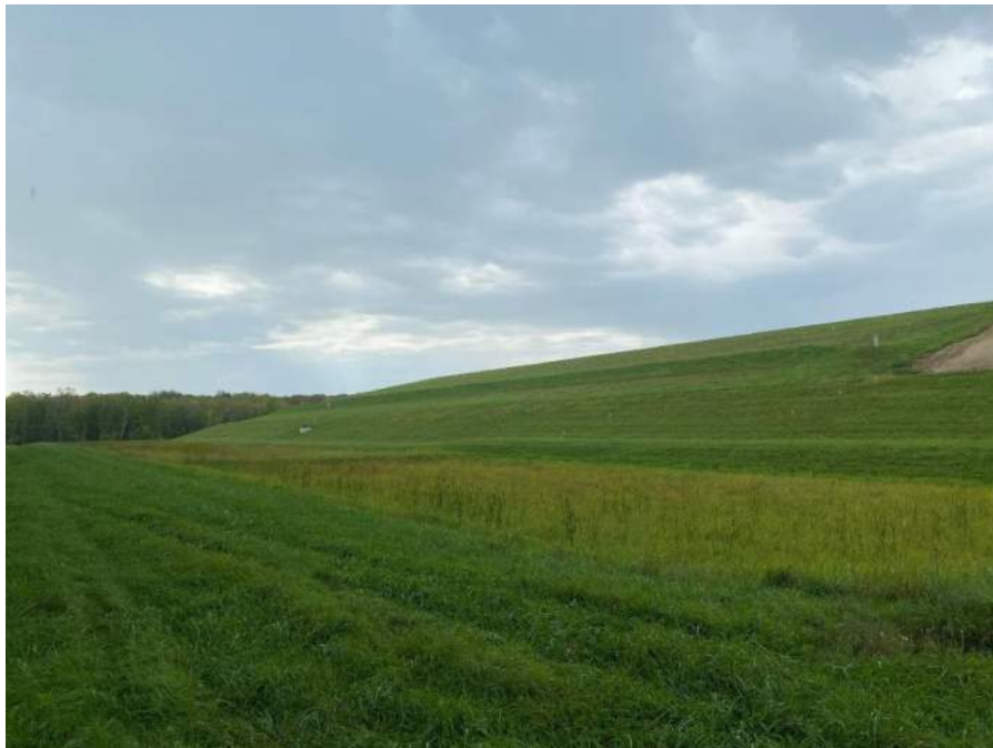
Photo No. 6 – Stormwater Basin 2 and Cell 2 final cover.
