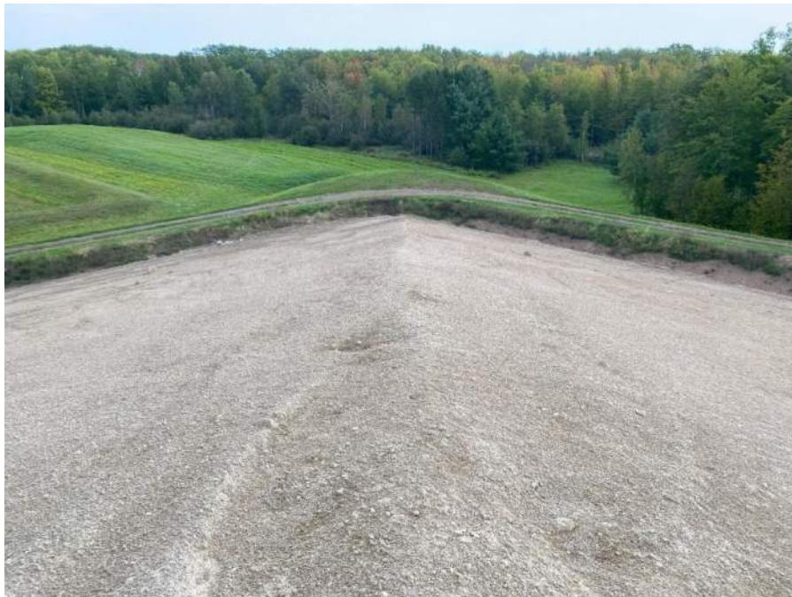
Photo No. 10 – Cell 1 north and east perimeter slopes, looking northeast.
