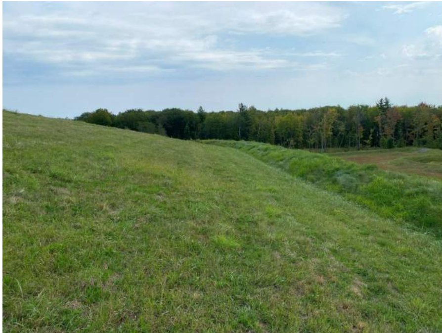
Photo No. 11 – Looking east at the Cell 2 east stormwater control ditch.
