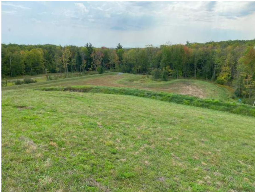
Photo No. 4 – Cell 2 south slope and stormwater diversion berm.
