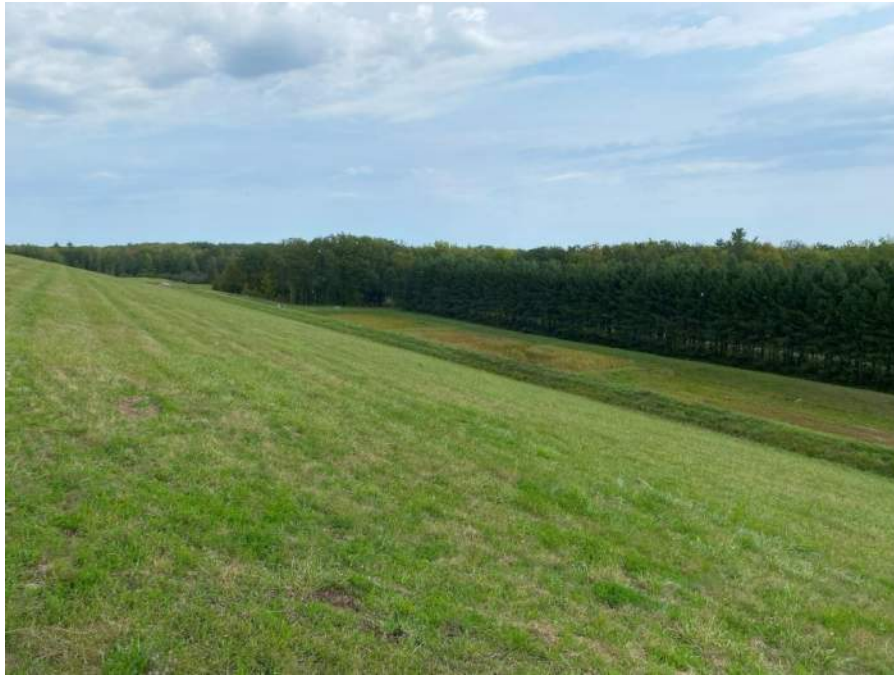
Photo No. 5 – Stormwater Basin 2 east of Cell 2.
