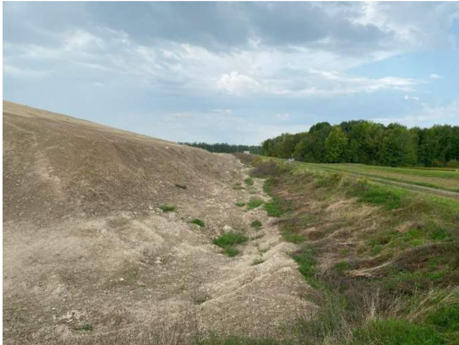
Photo No. 9 – Looking west at the Cell 1 north perimeter slope and leachate collection ditch.
