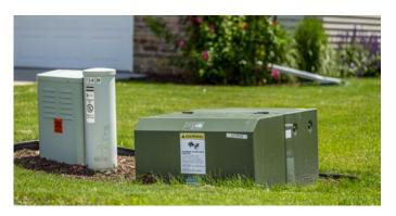
**Look around.** Be sure not to block pad-mounted equipment, natural gas or electrical meters, well heads, or cable TV boxes with your new construction. Pools or decks too close to utility equipment could be damaged during required repairs and could delay service restoration. Obstructions should not be placed within 10 feet of this type of equipment.
